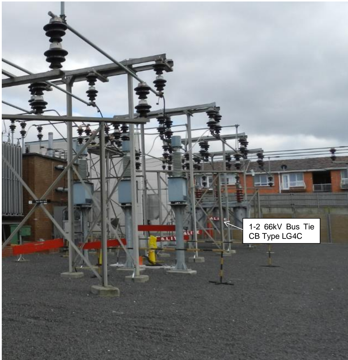
Figure 2-4: FE 66kV Bus Tie CB and 66kV insulators
