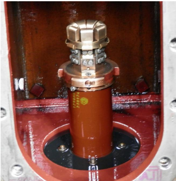
Picture 4: New fixed contact installed on white phase of FDR FW13 22kV CB
