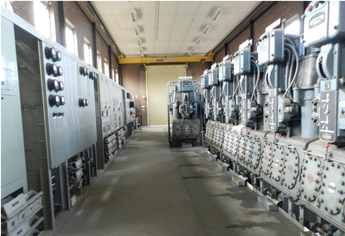
Figure 2-3: FE 22kV Switchgear
