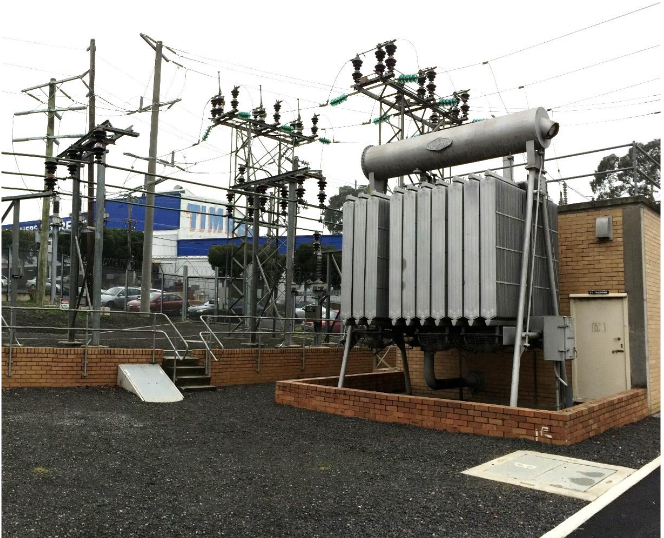
Figure 2–3: HB Transformer Enclosure, Radiator and 66kV Bus
