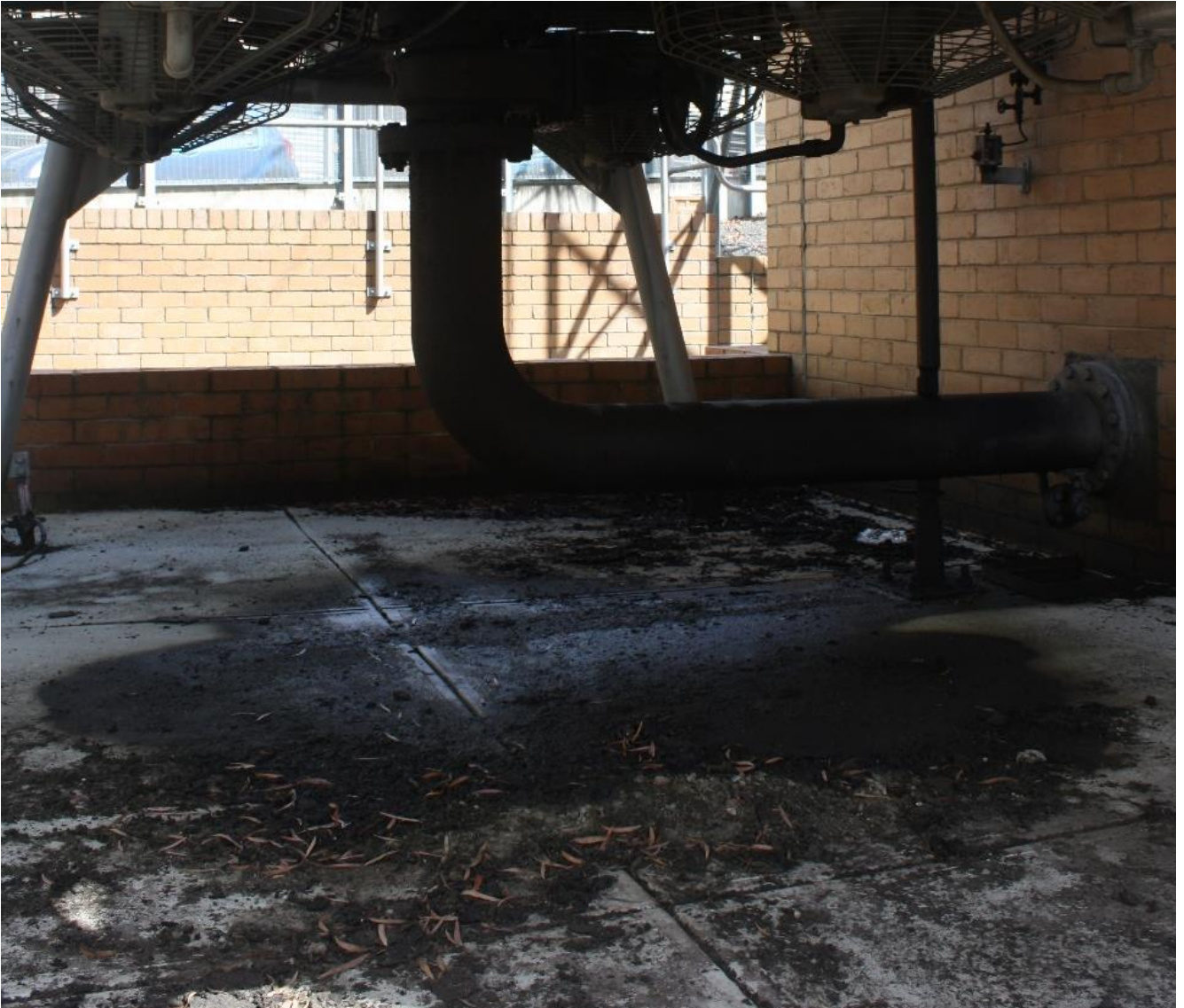
Figure 2–4: HB No.1 Power Transformer Radiator Oil Leaks
