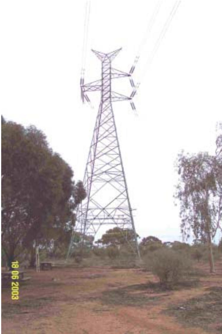
220kV, Single Circuit Strain Tower
