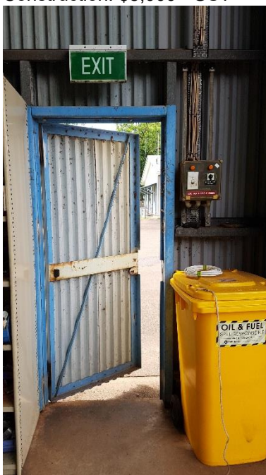
Photo 1. Existing Pedestrian Door 1
