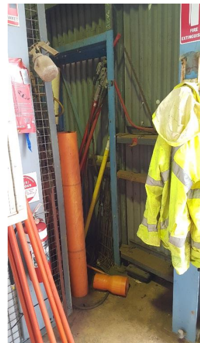
Photo 3. Blocked Pedestrian Door 2
