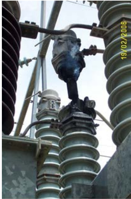
Figure 2 – Failed HLC circuit breaker at Snell Street zone substation
