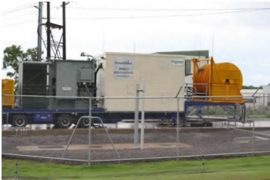
Figure 1: NOMAD Modular substation located at Wishart
