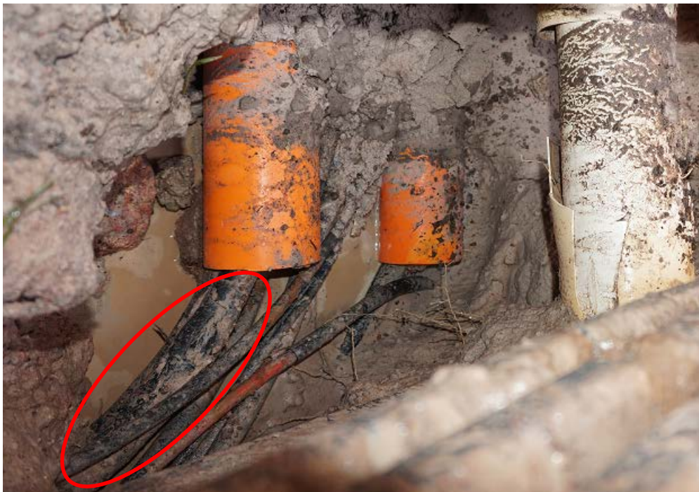
Figure 2 – Cable inspected prior to failure
