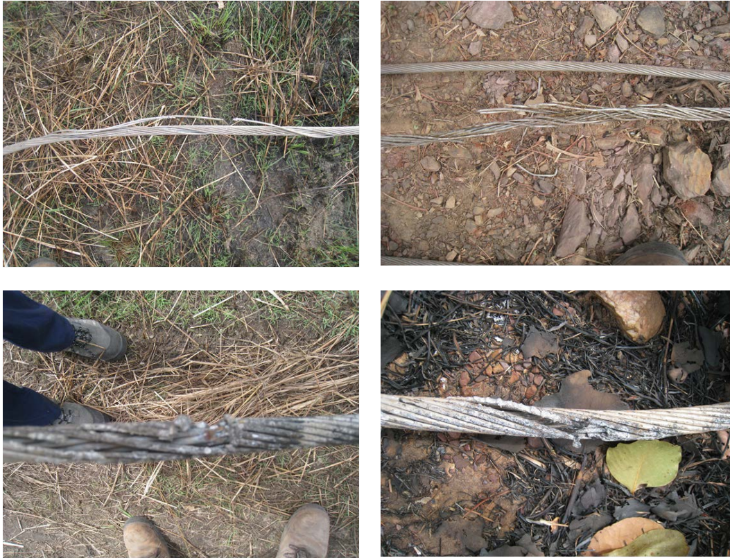
Figure 1 – Cockatoo conductor photos showing broken strands, burning and corrosion
