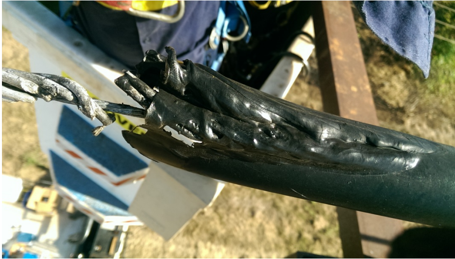
Figure 2 – Damaged conductor Due to “poly-pipe” bat guards
