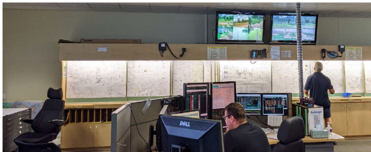
Figure 4 – Power and Water pin boards for distribution management
