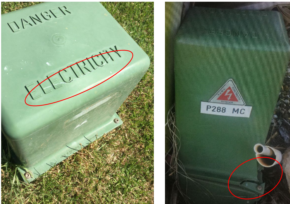
Figure 12 Cracks in the pillar cover
