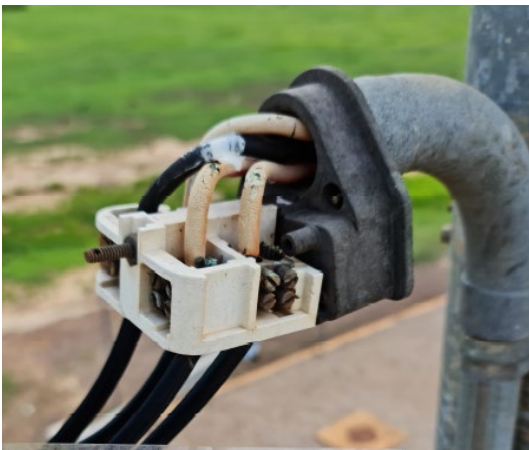
Figure 11 Common defects at Point of Attachment
