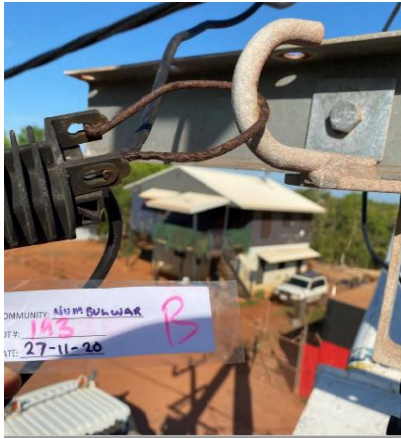
Figure 10 Service clamp defects
