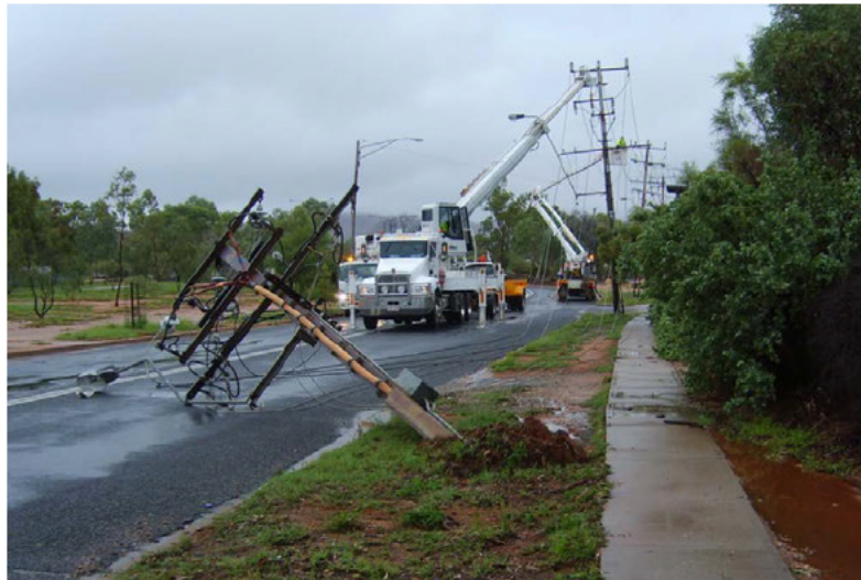
Figure 1 Undoolya Rd Pole Failure 10/01/2015 Due to Footing Corrosion
