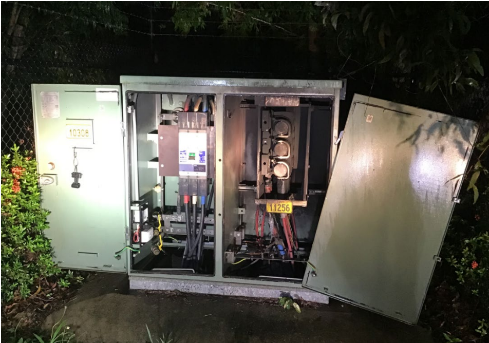
Figure 2 Photo of switchgear enclosure following explosive failure (DT2850)
