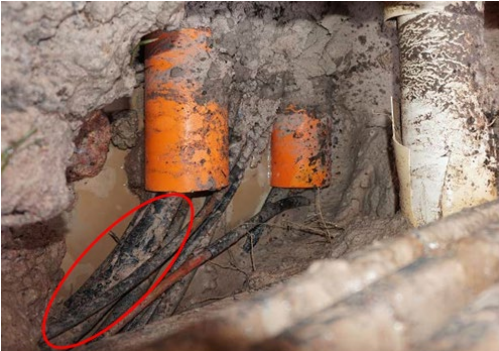
Figure 7 Cable inspected prior to failure
