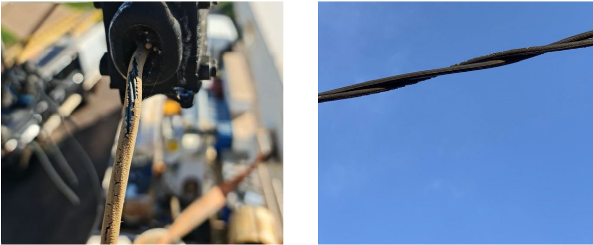
Figure 8 Insulation damage exposing conductors
