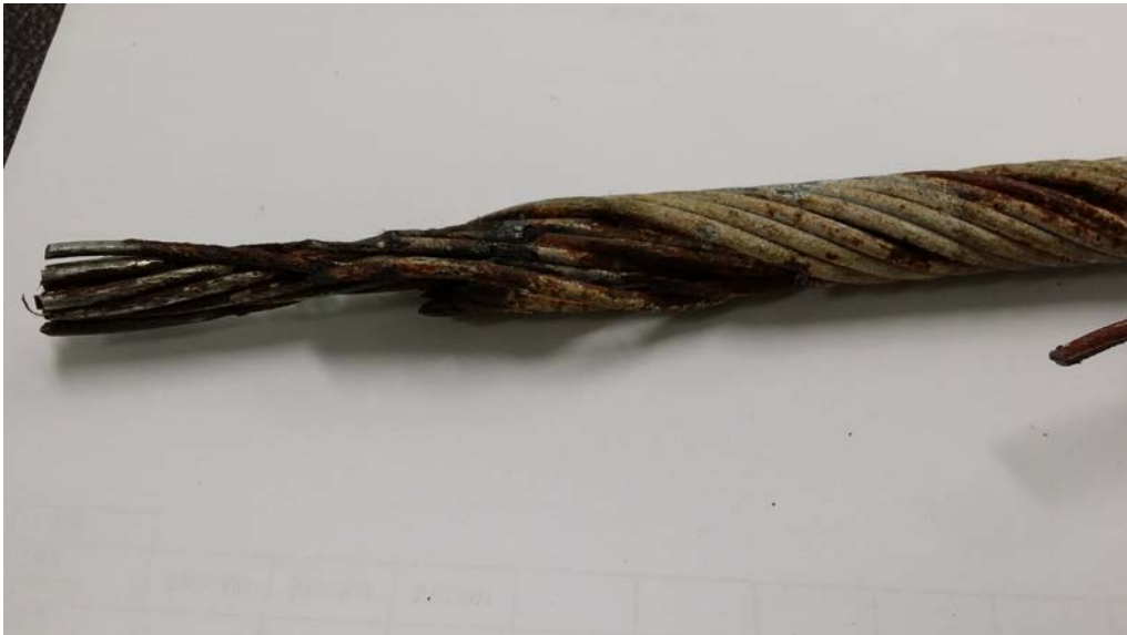
Figure 3.20: Example of conductor corrosion and lightning damage from NT network
