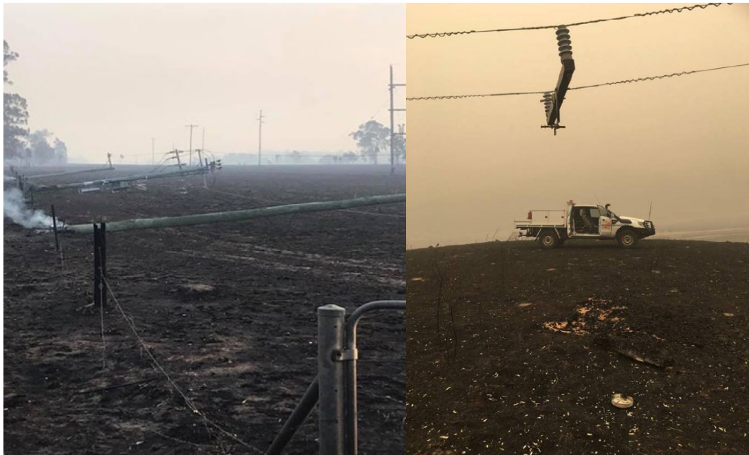
Figure 3 – Left: Timber CCA poles 2019/20 bushfires. Right: Timber pole burnt away, only composite cross arm remaining
