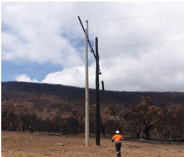
Figure 1 - Adjacent composite and timber CCA poles exposed to bushfire
