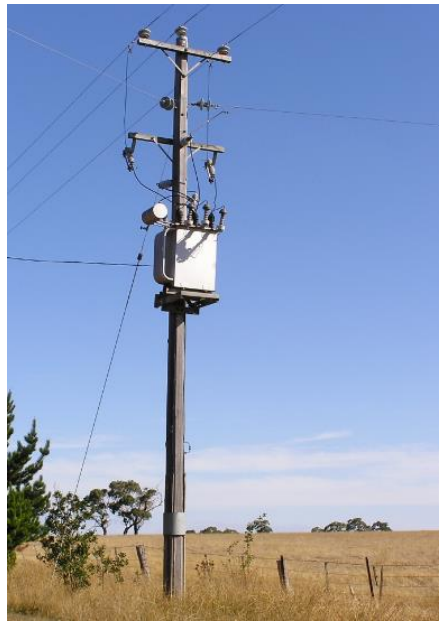
Figure 1-9 – Picture of a typical pole mounted distribution substation
