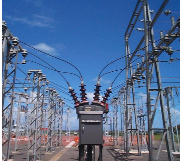
Figure 1-10 – Picture of a Circuit Breaker within a Zone Substation
