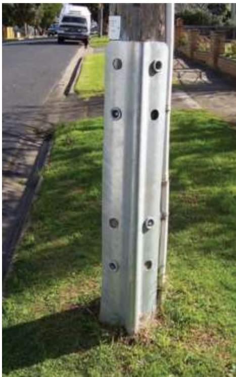
Figure 36: example of [REDACTED] RFD Pole Reinstatement 182
