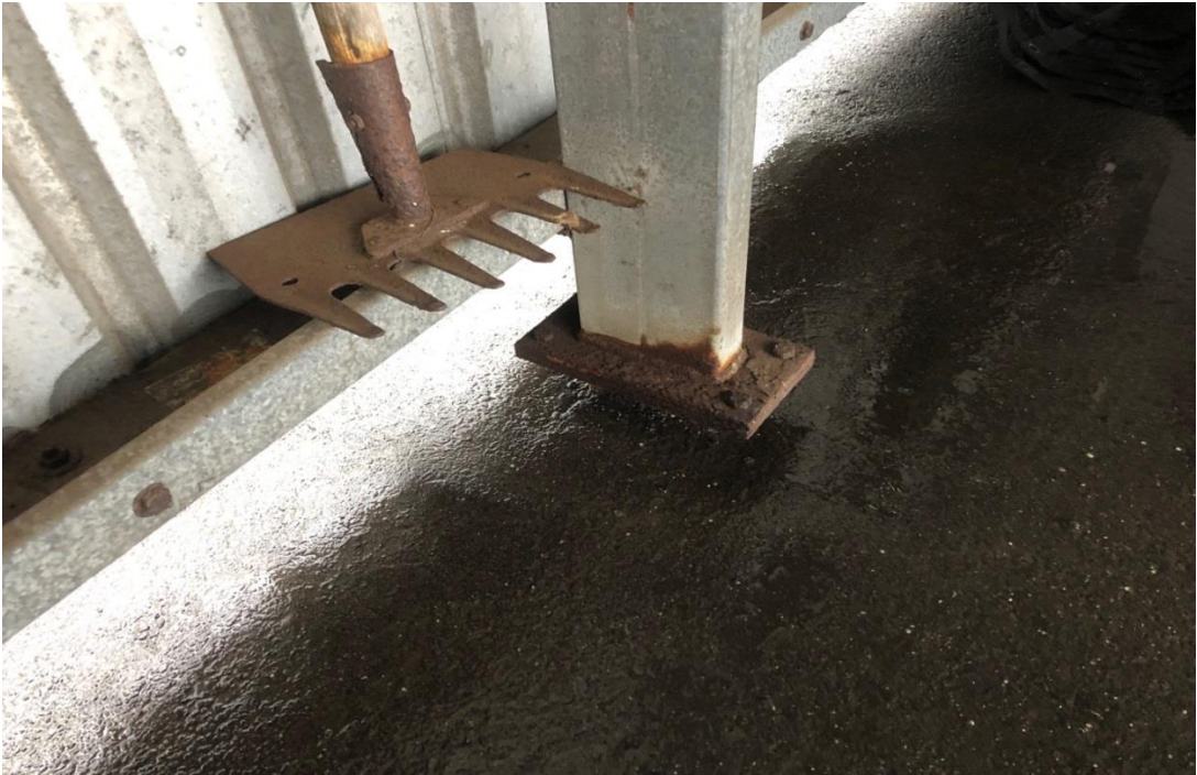
The frame footing of the trailer shed.
