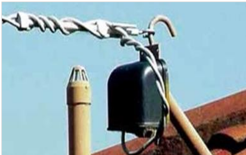
Figure 4.5 Sample image: twisted PVC service line
