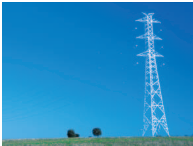
A 330kV transmission tower at Kindon Station, Millmerran.
