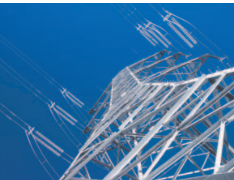
A transmission tower on Kindon Station, Millmerran.
