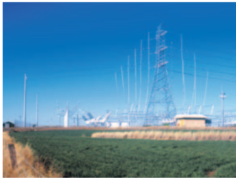
Powerlink has regimes in place to monitor compliance with environmental regulations (Millmerran substation).
