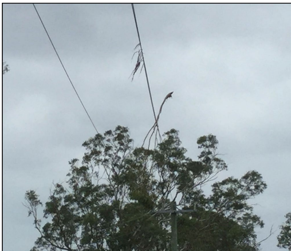
Figure 2 – Vegetations fallen across the wire INCD-2095253-a
