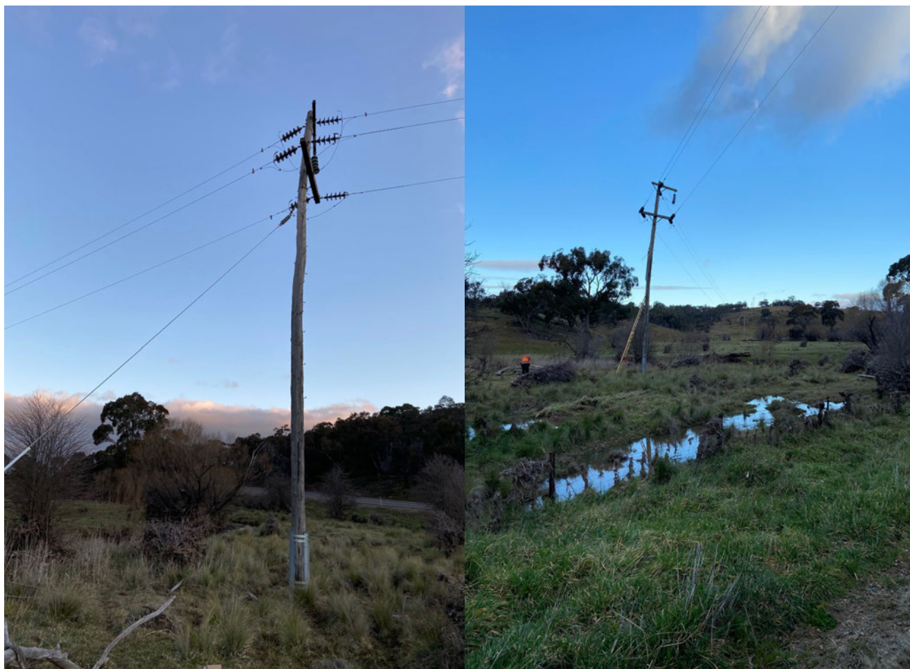
Figure 5 – Example of poles in swampy areas
