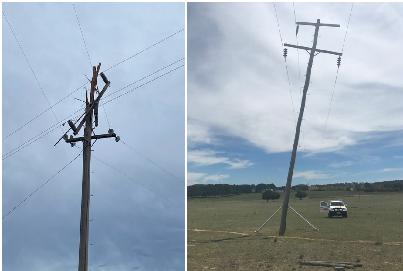
Figure 4 – Poles damaged by lightning and by high winds
