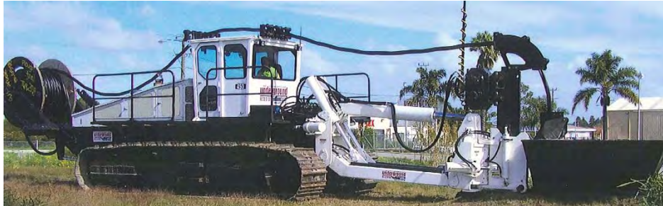
Figure 20: Plough for undergrounding cable
