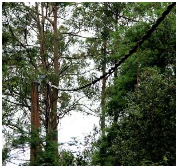
Figure 21: Typical high voltage ABC powerline in a heavily forested area
