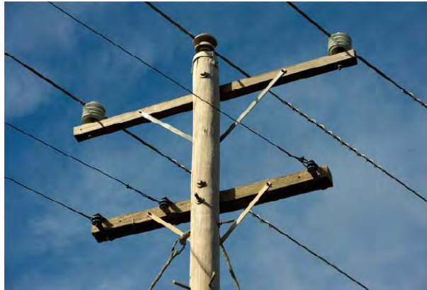
Figure 18: Power pole with high voltage lines at the top of the pole and low voltage lines underneath
