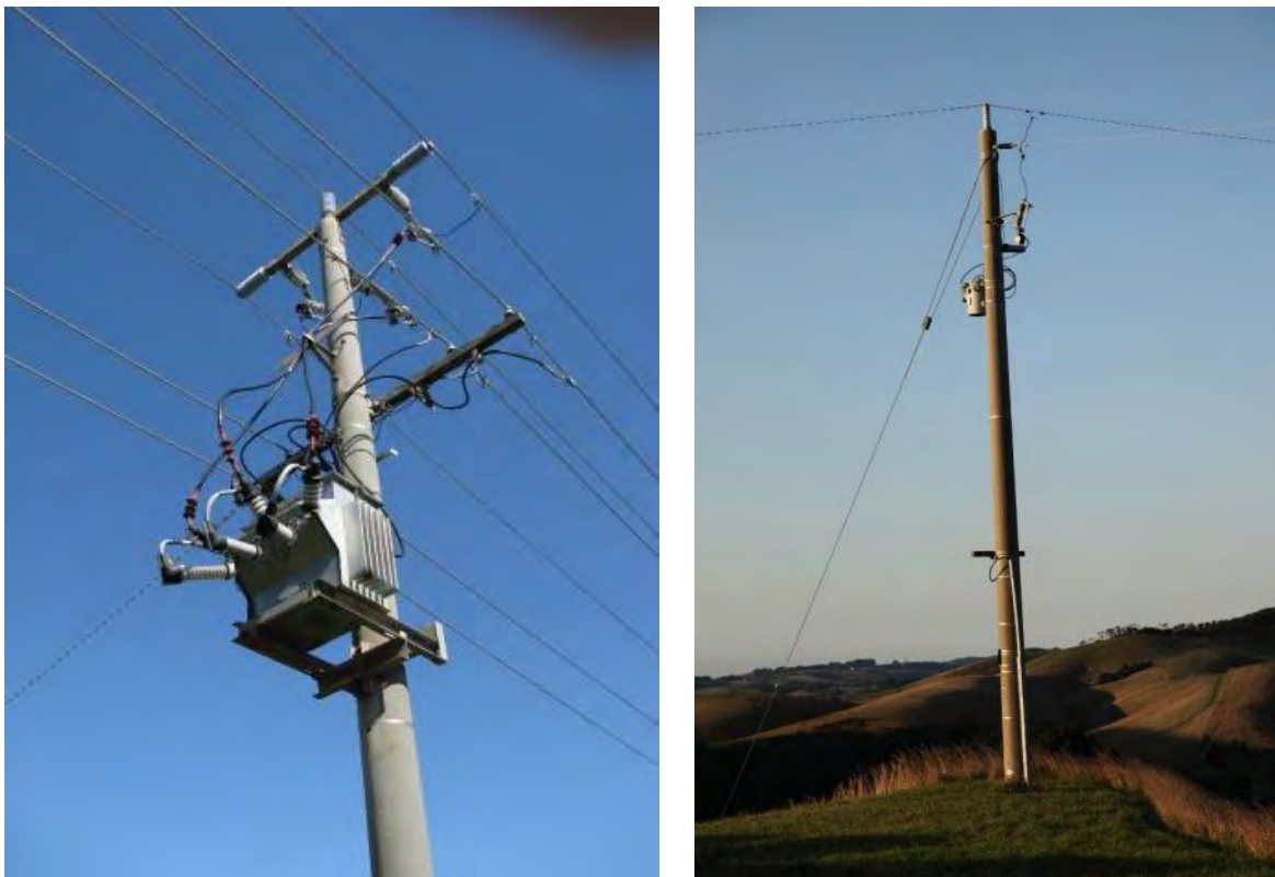
Figure 2: Examples of multi-wire high voltage distribution line (on the left) and SWER line (on the right) Distribution and SWER powerlines in rural areas were the focus of the Royal Commission's recommendations.
