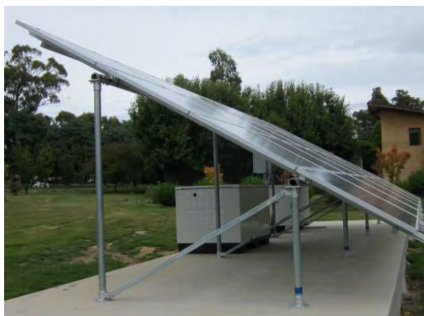
Figure 29: SAPS installed for one participant in the Taskforce’s trial
