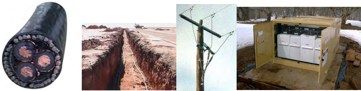
Figure 19: Typical high voltage underground cable, installation trench, termination structure to connect to overhead lines, and ground level auxiliary equipment associated with underground cable
