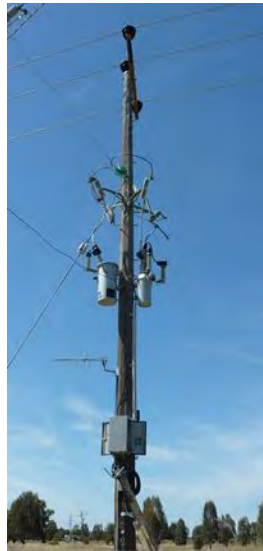
Figure 14: New generation SWER ACR (pictured on the right hand side of the pole)
