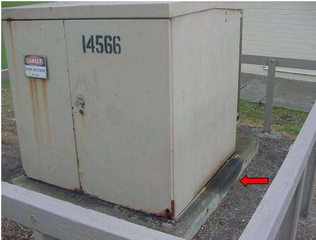
Example of P1 – Oil on ground
