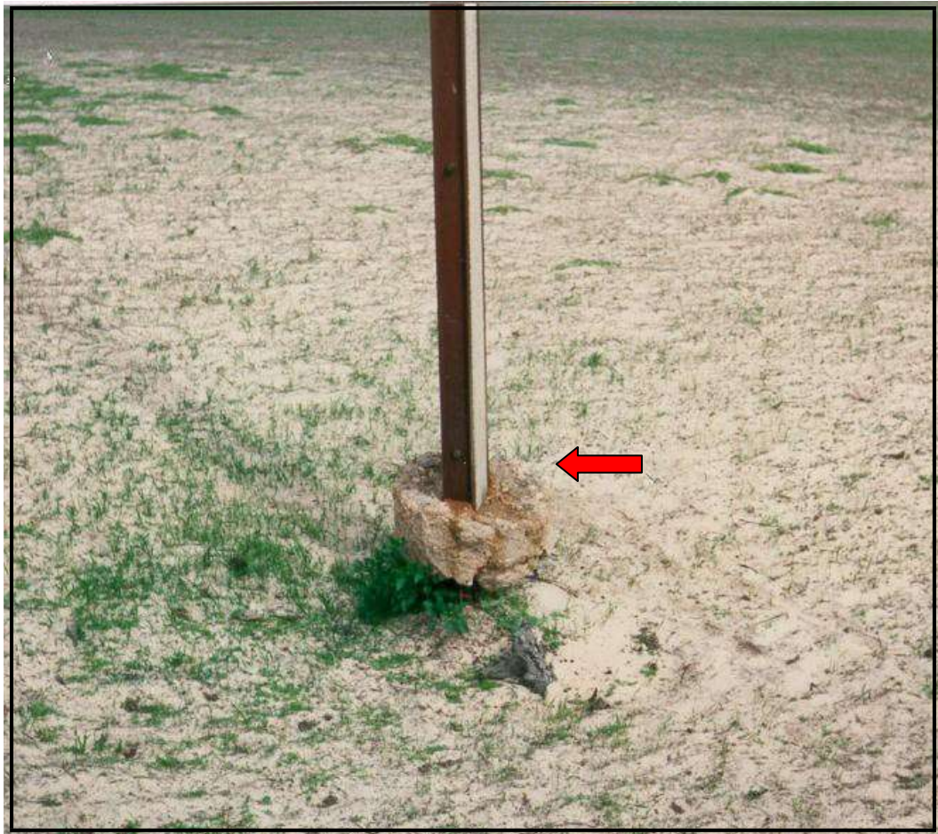
This photo is typical of P1 defect
