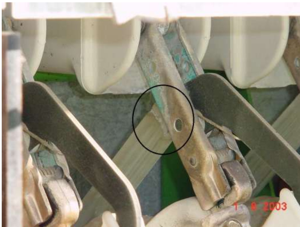
This photo is typical of P2 and fail cubicle for live operation
