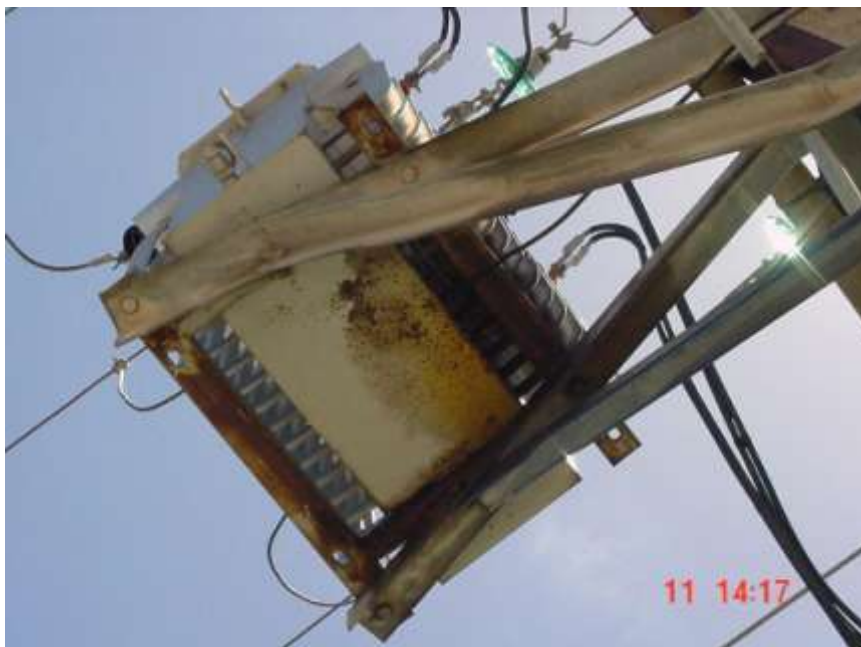
Examples of Transformer Oil Leaks
