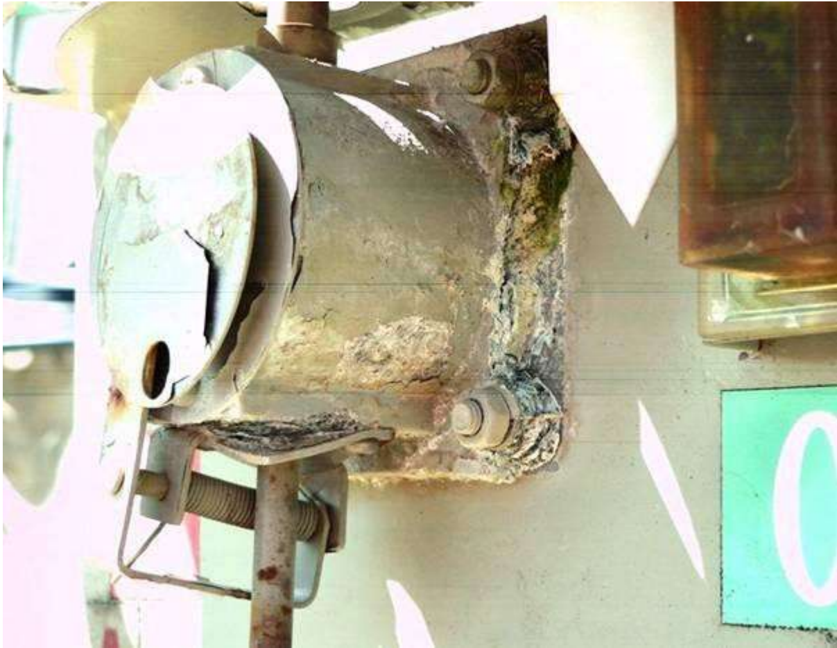
Example of Priority Breakdown as the gas will have dispersed (failed unit).
