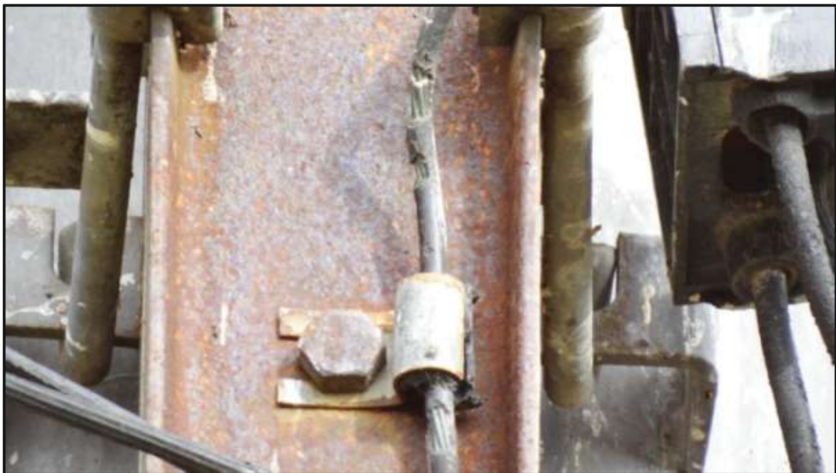
Note: This does not require to be recorded as a defect
