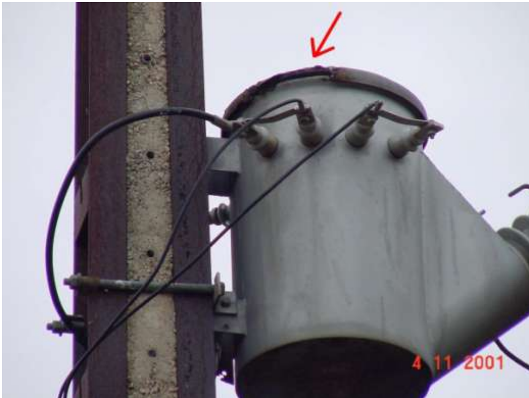
Example of Transformer Corrosion – Priority 1
