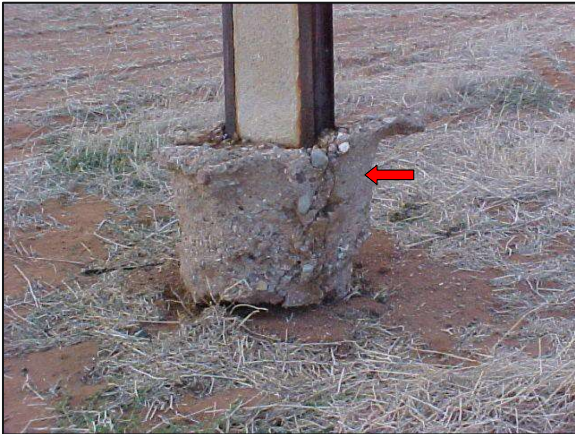
This photo is typical of P1 defect
