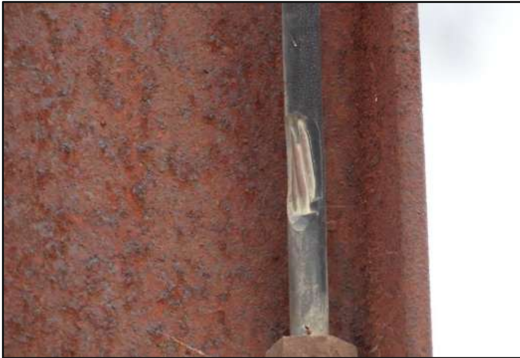
Note: This does not require to be recorded as a defect
