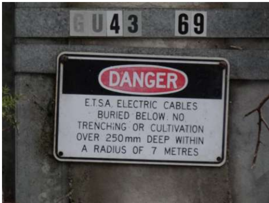
Examples of 11kV/7.6kV/33kV TFs warning signs.
