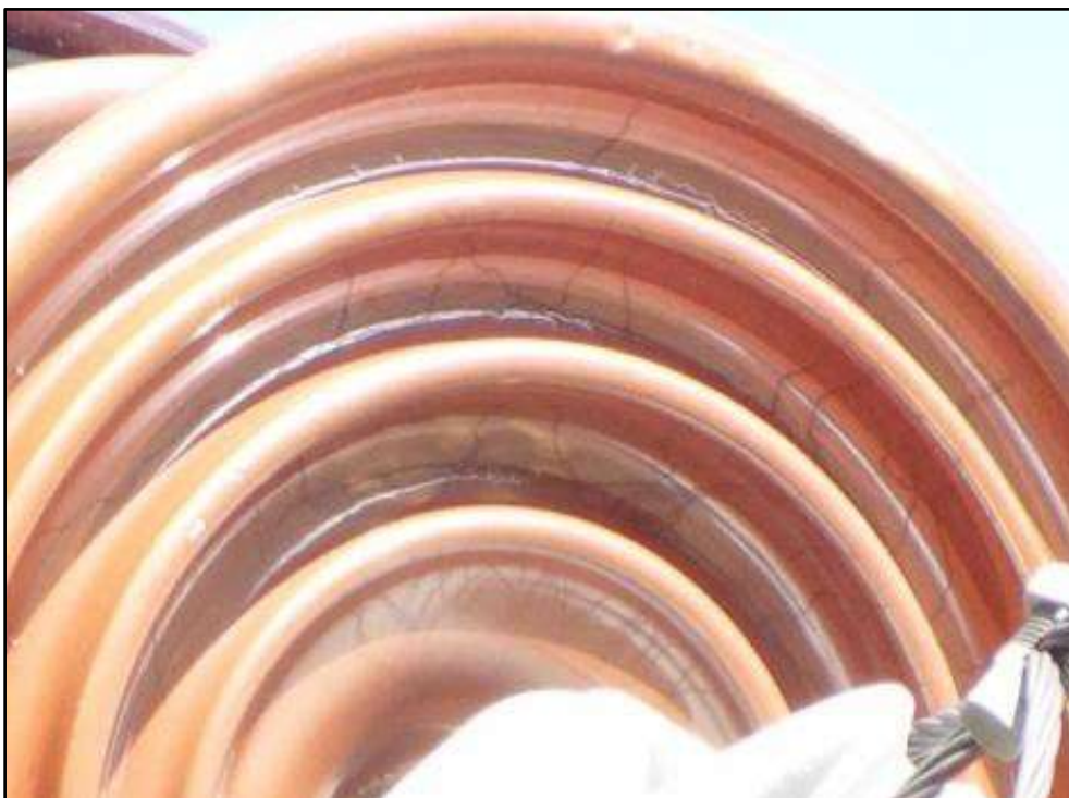
Note: This does not require to be recorded as defect
