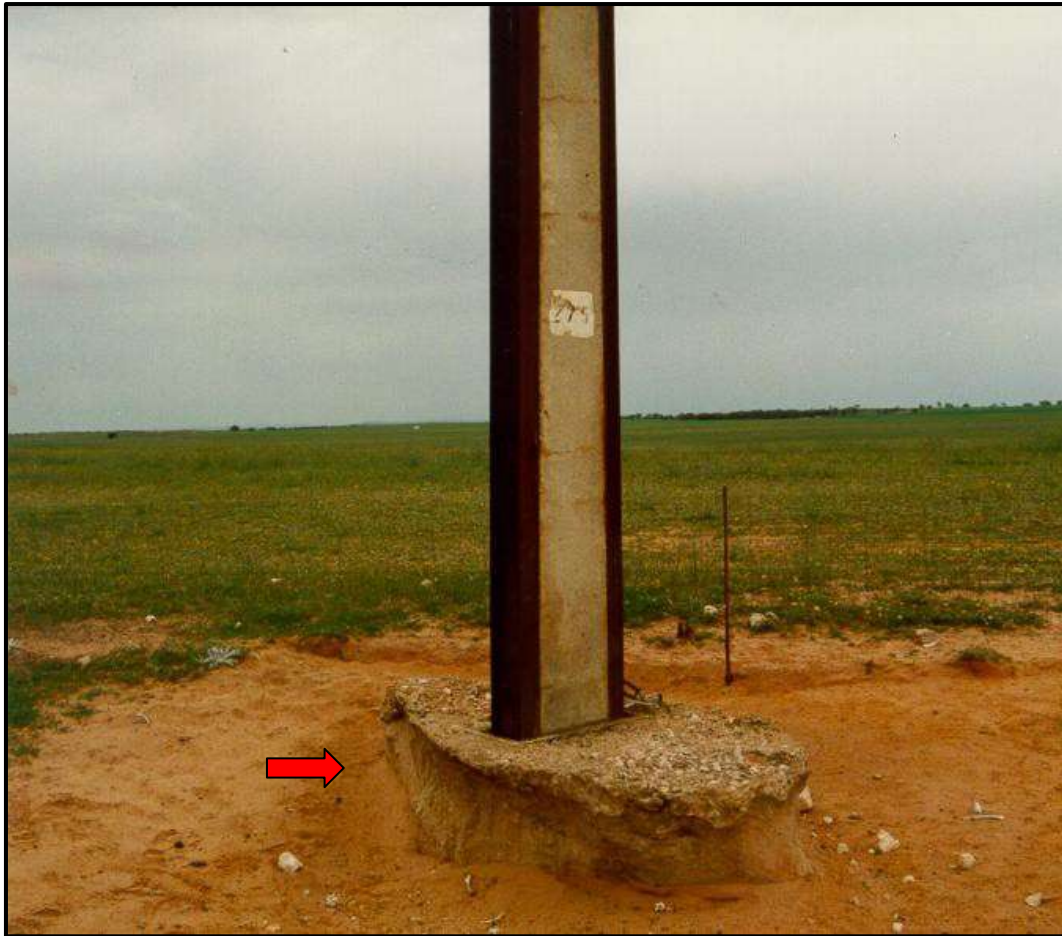
This photo is typical of P2 defect
