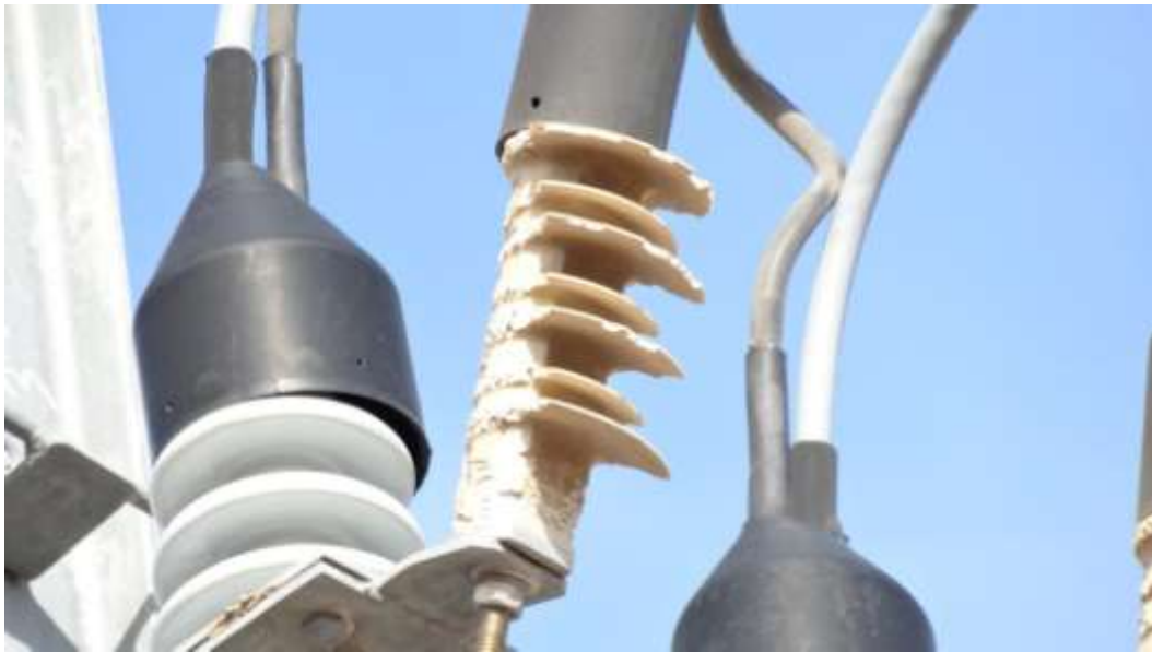
This photo is an example of P1, damaged surge diverters
