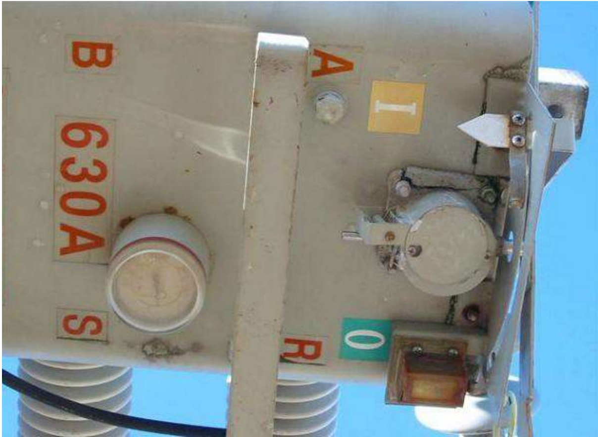
Example of P1 due to significant cracked housing.
