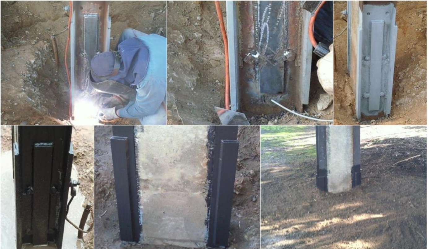
Figure 4: Pole Plating being undertaken
