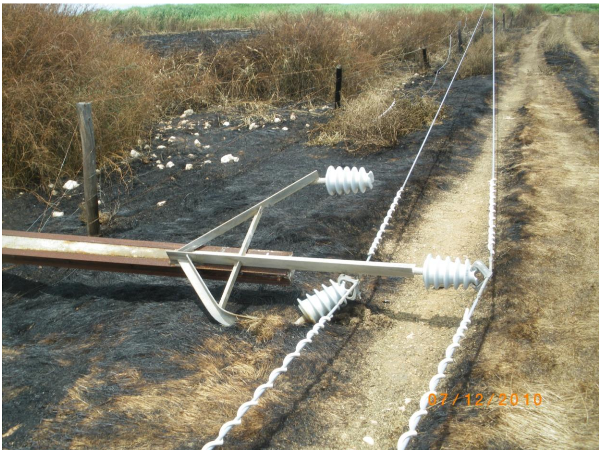
Figure 5: Fire Started by pole failure - ST22 Bagley Bridge 11kV Feeder
