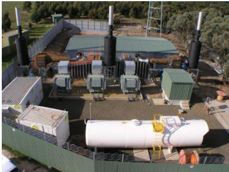
Figure 5: Construction of 6MW of generation at Kingscote
