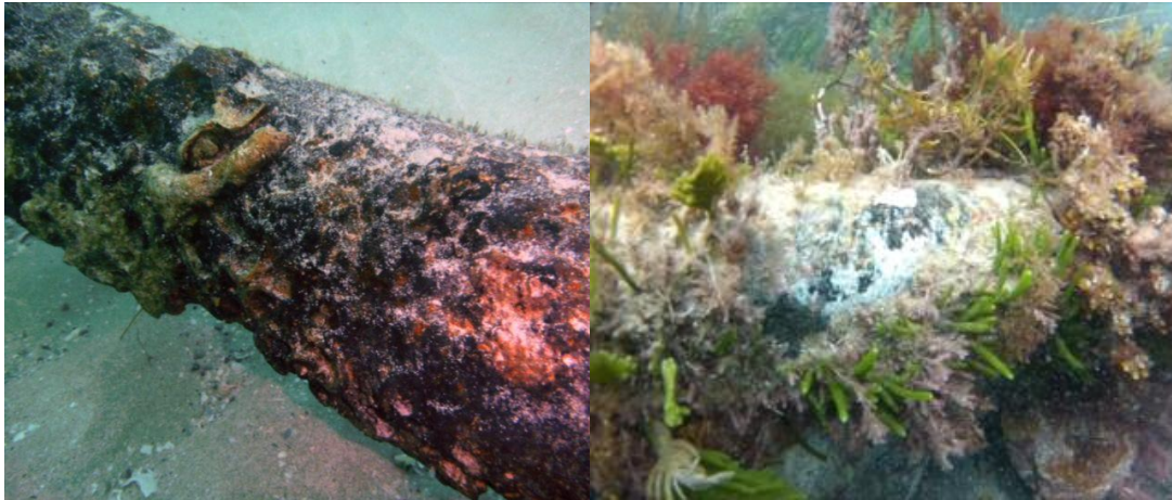
Figure 3: Underwater inspection showing minor corrosion on existing submarine cable
