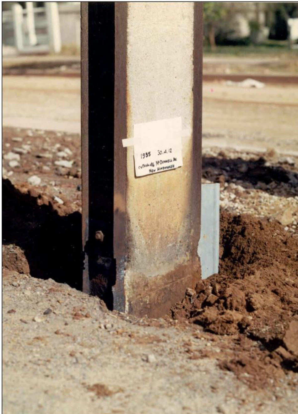
Figure 11: Stobie pole ground level corrosion example
