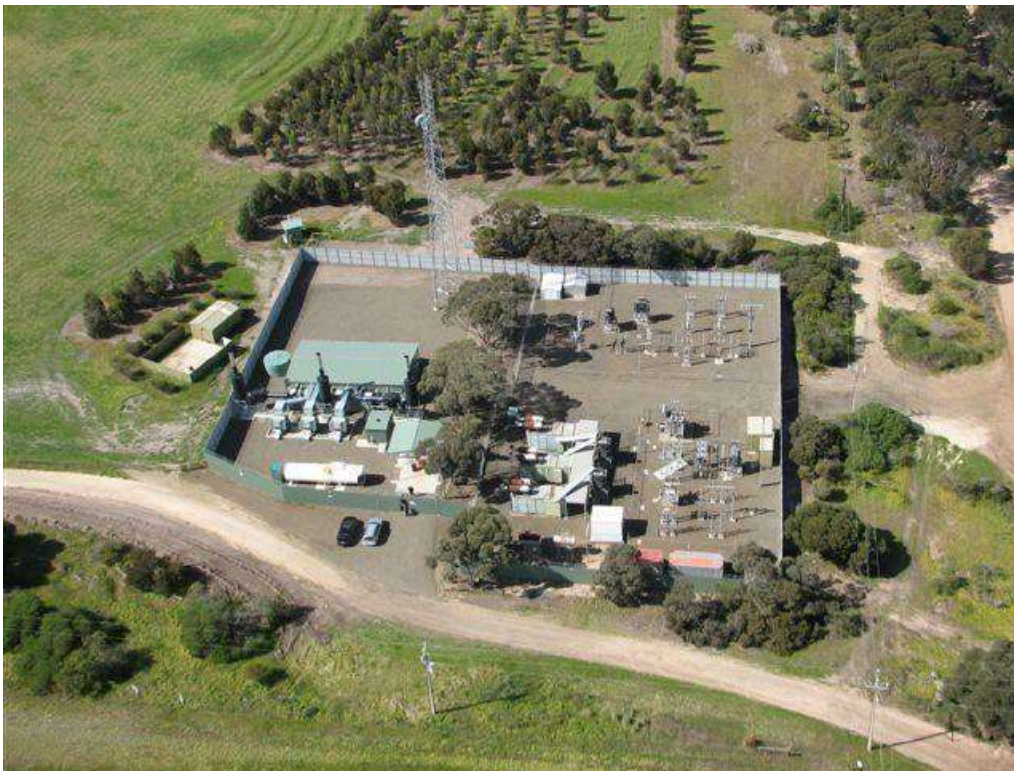
Kingscote Substation and Kingscote Power Station to left
