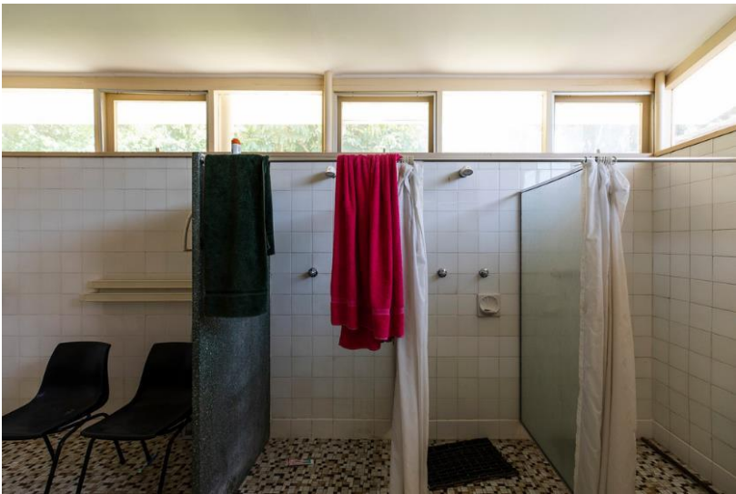
Figure 24 Pole construction showers all in very poor condition and original fit-out
