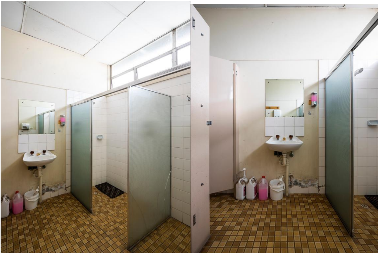
Figure 21 Toilet and shower cubicles all original 1950's fit-out in very poor condition.
