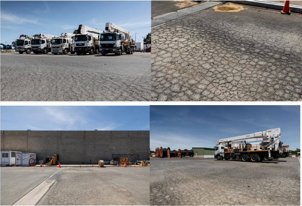
Figure 10 Examples of significant bitumen damage to semi-trailer route and turning circles and Transmission Heavy Vehicle Parking and Storage areas
