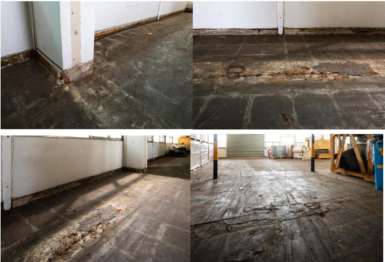
Figure 19 Example of extensive floor cracking, rising damp and concrete cancer throughout interior of the old admin building.
