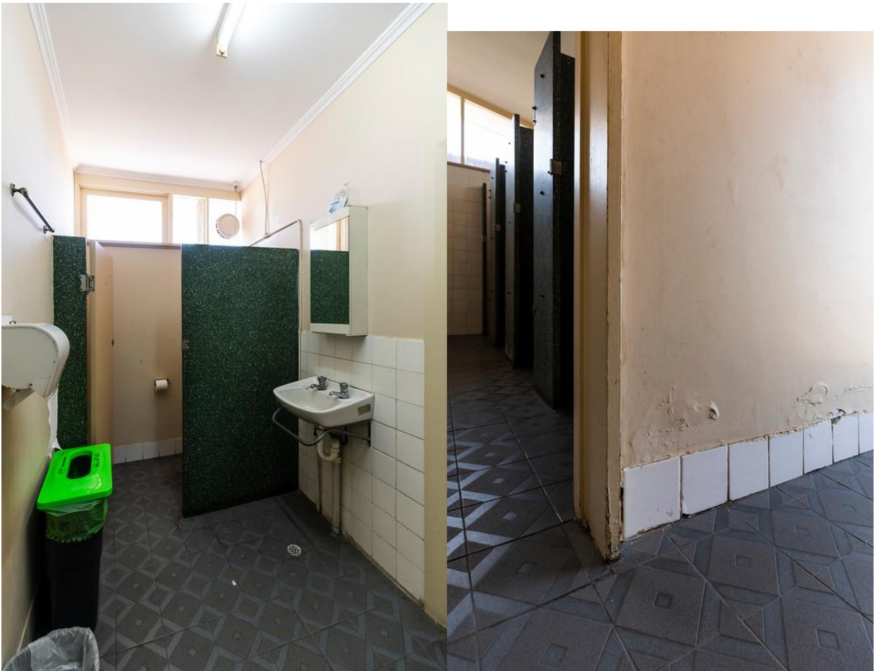
Figure 26 Pole Construction Ladies Toilet – No Female Shower, rising damp and concrete degradation
