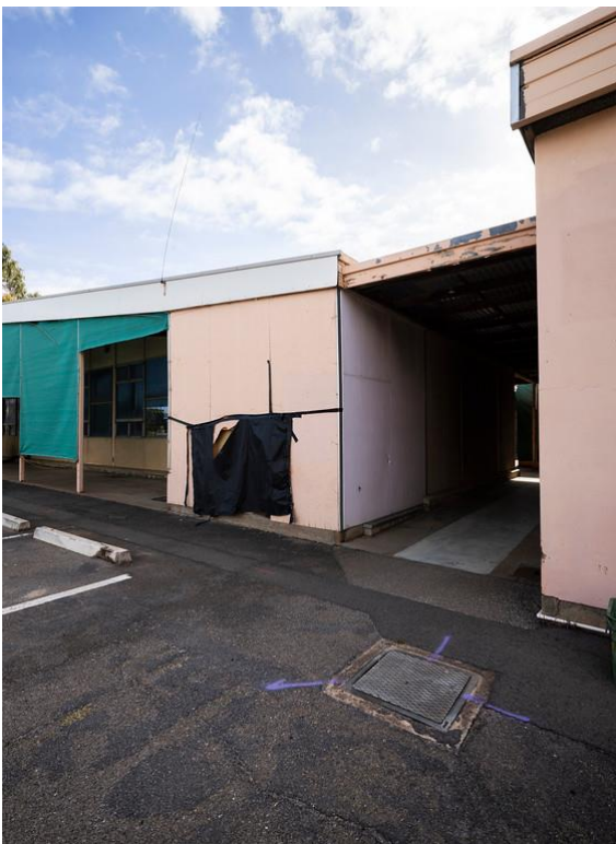
Figure 14 Cement fibre cladding in various states of rot and disrepair and damage.
