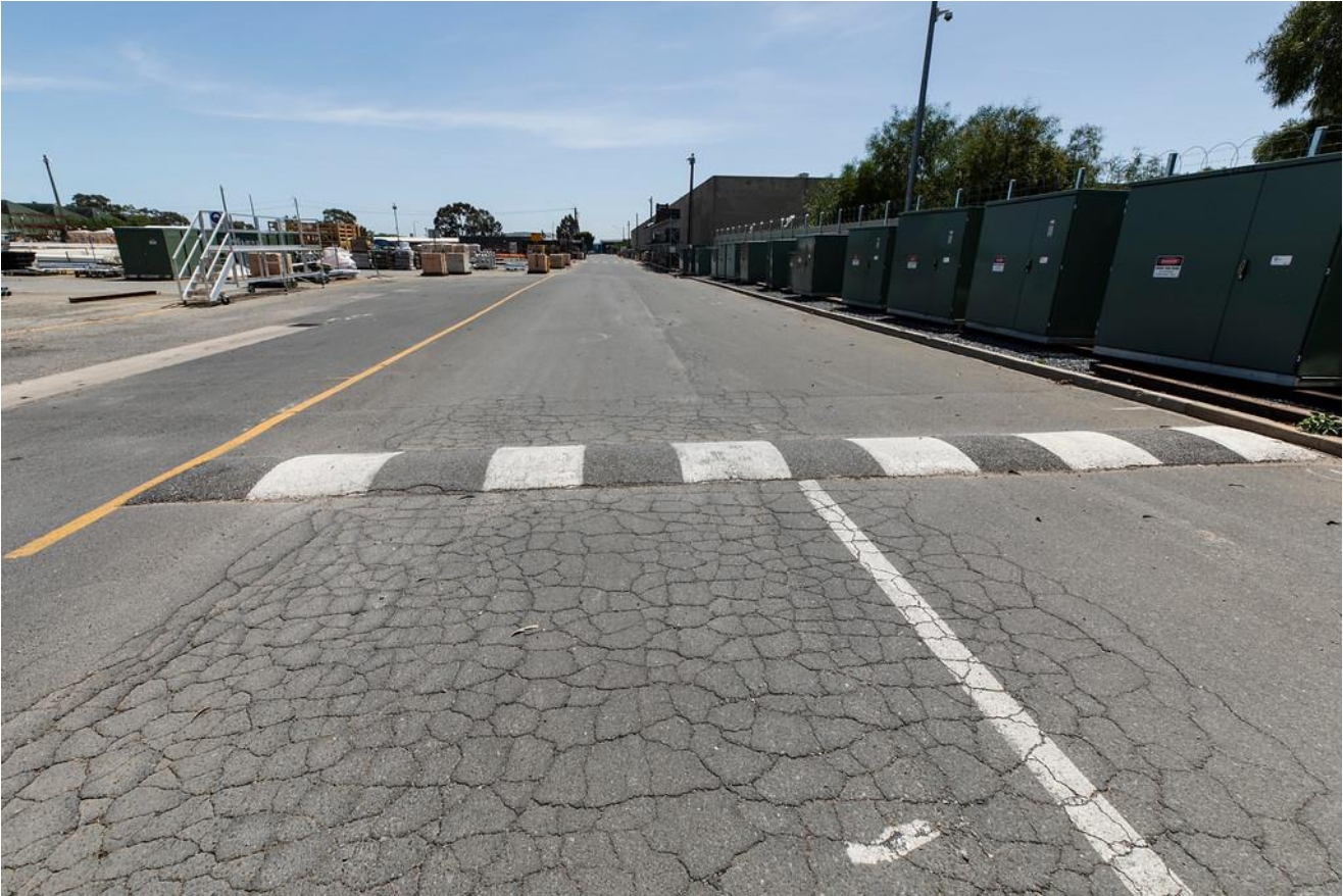
Figure 9 Example of significant full-thickness crack and subsidence to main driveway route for heavy vehicles.
