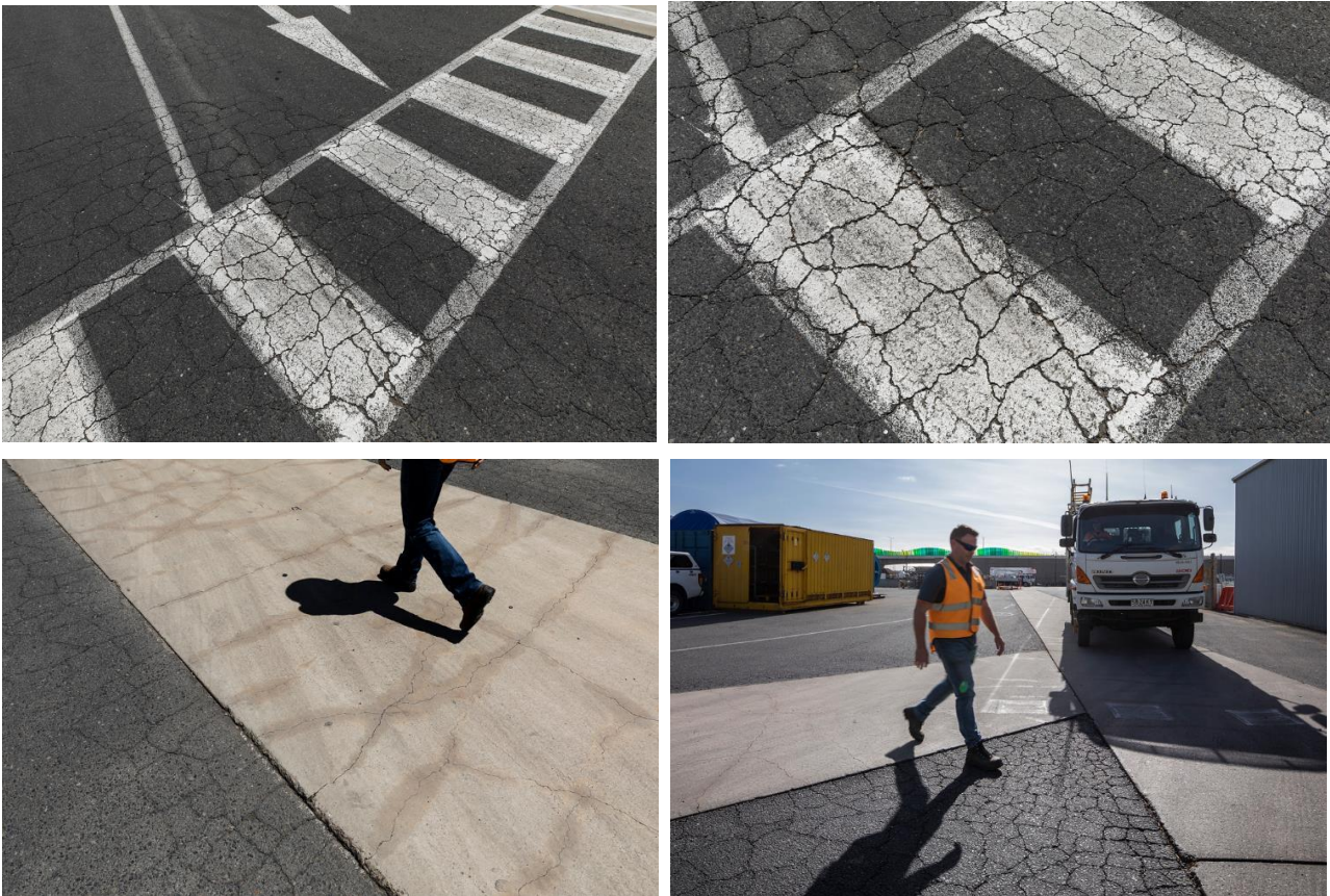
Figure 11 Examples of cracking and damage to pedestrian walkways, thoroughfares and concrete drainage areas. Also showing previous glue repair failures.
