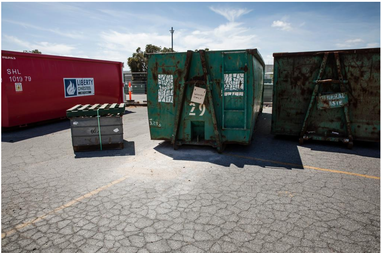
Figure 7 Example of extensive full-thickness bitumen cracking to salvage bin storage, loading and unloading areas (9m storage bins can be over 3 tonne in weight).
