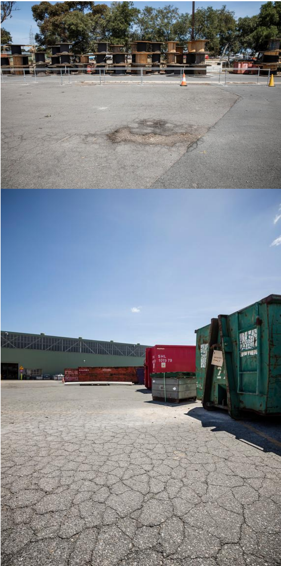
Figure 8 Further examples of cracking and potholing and subsidence of sub-grade to logistics salvage area.
