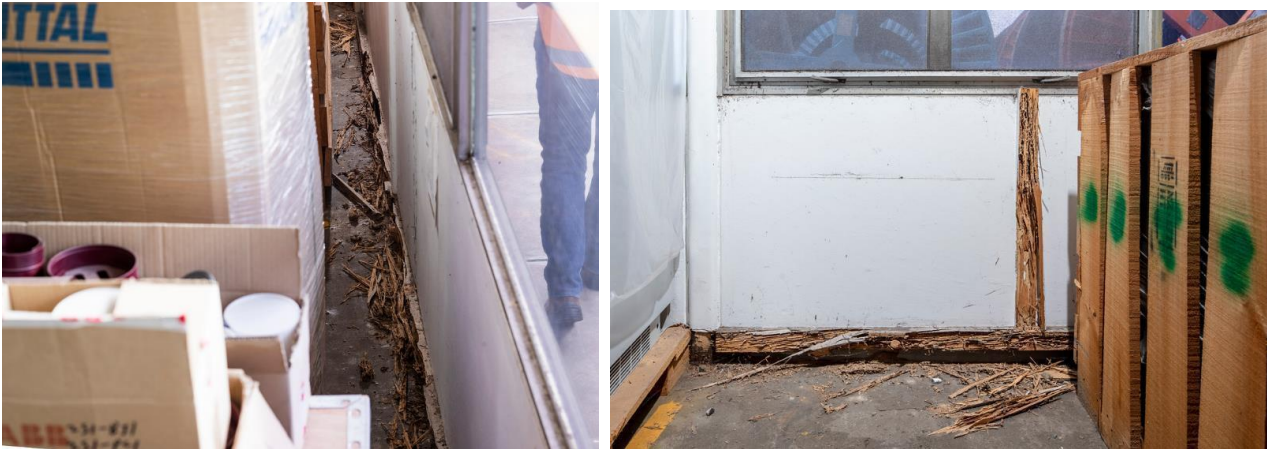
Figure 18 Example of significant termite damage to internal timberwork in old admin building.
