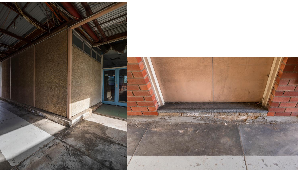
Figure 16 Examples of extensive rising damp and concrete cancer to wall foundations and damage to amenities block brick work and foundations
