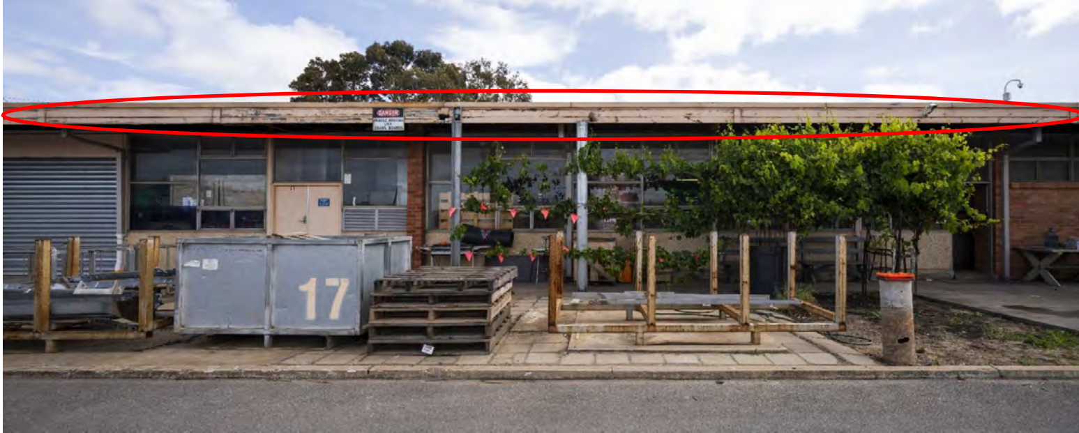
Southern side of the old Admin building – timber fascia rot and degradation
