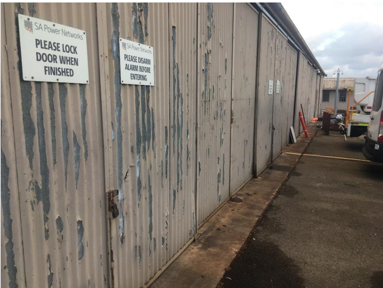
Figure 12 Examples poor condition of corrugated iron sheets of shed/workshops
