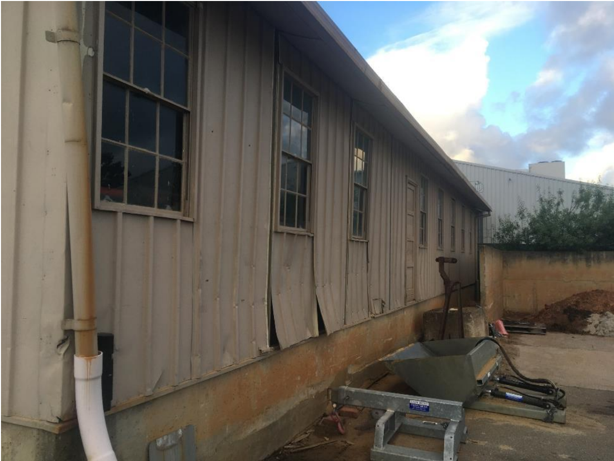
Figure 13 Examples poor condition of corrugated iron sheets of shed/workshops
