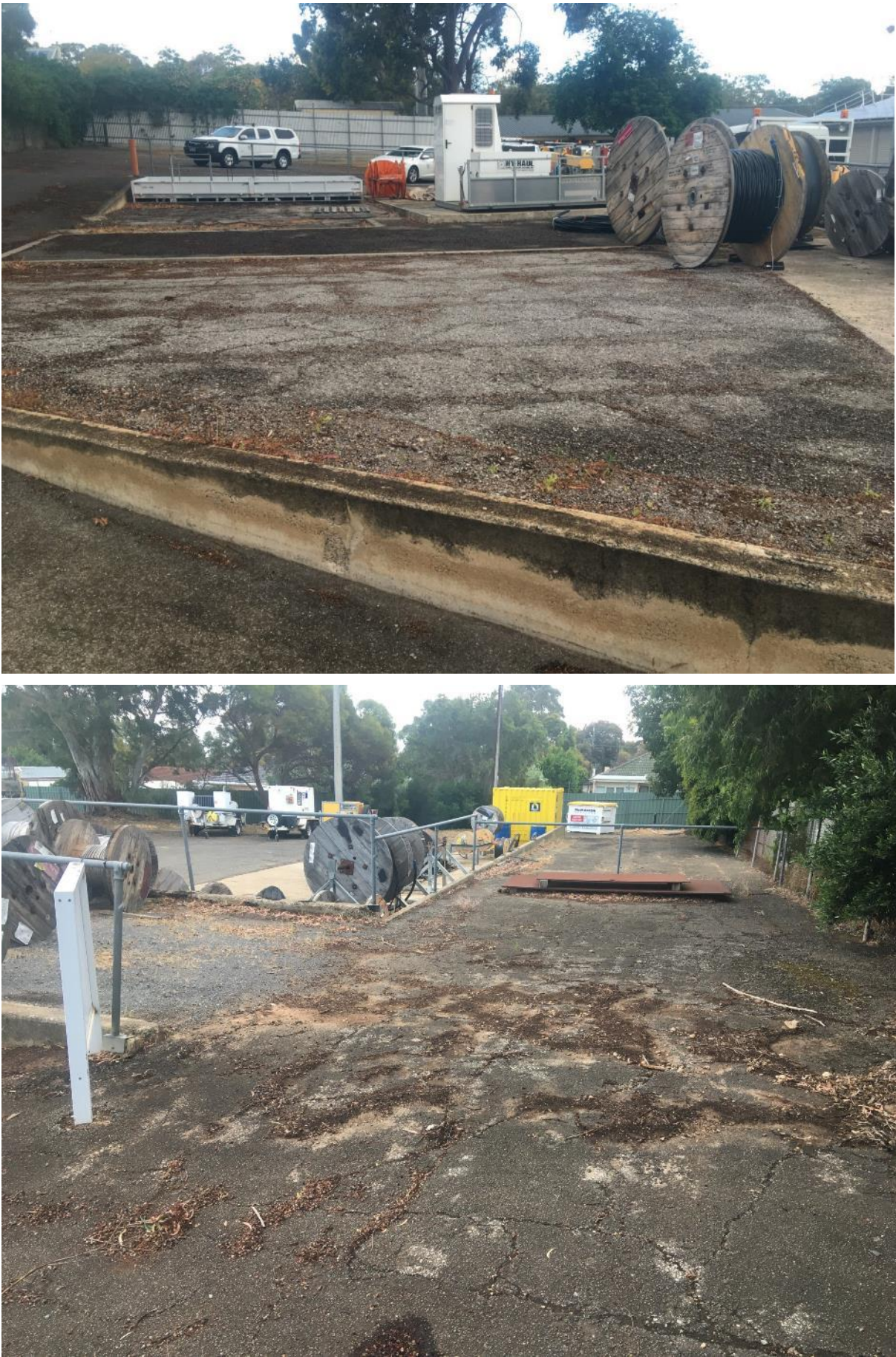
Figure 10 Examples of cracking, subsidence and tree root uplift to storage areas.
