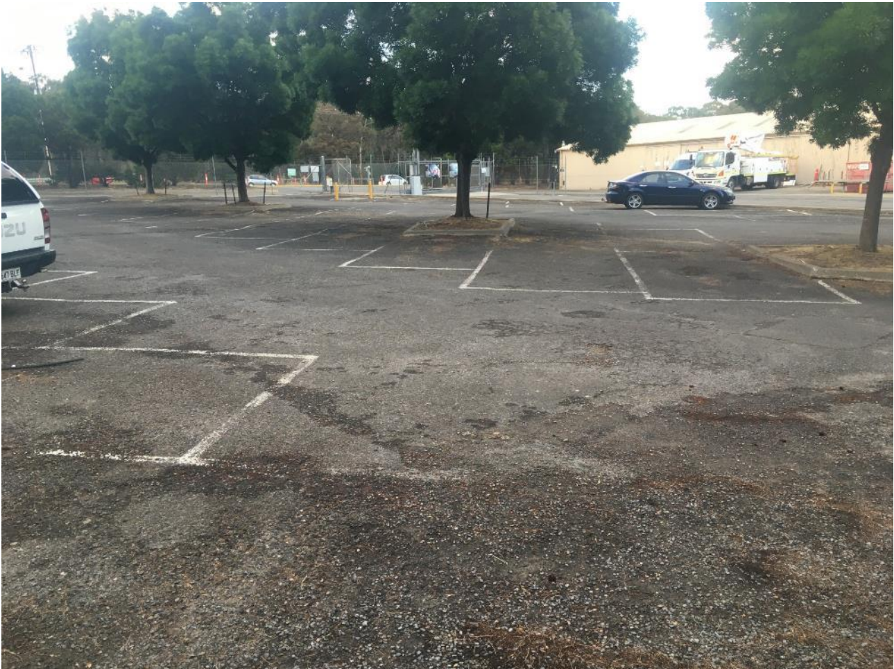
Figure 6 Example of complete breakdown of some areas of bitumen to the light vehicle car park and driveways.
