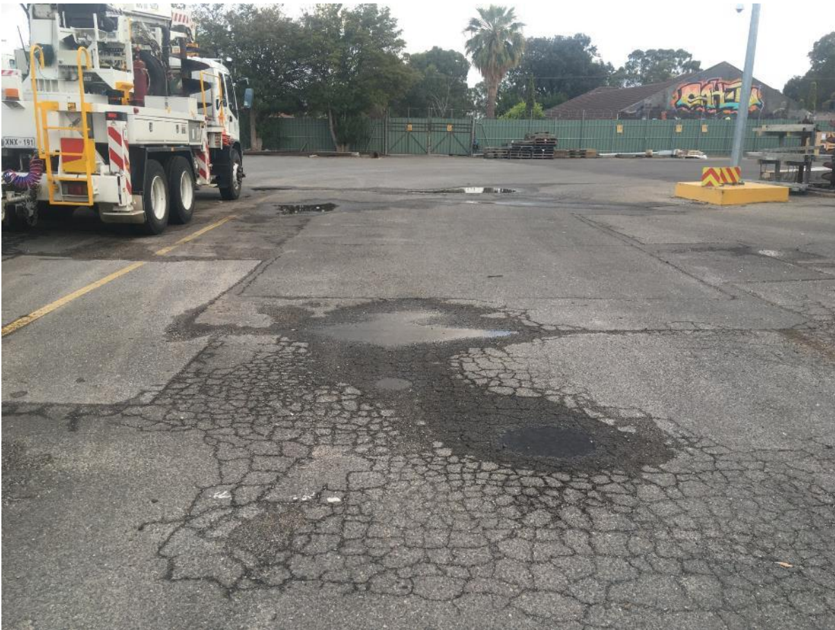
Figure 8 Example of full-thickness cracking, potholes and subsidence to heavy vehicle driveway. Also areas of previous repairs.
