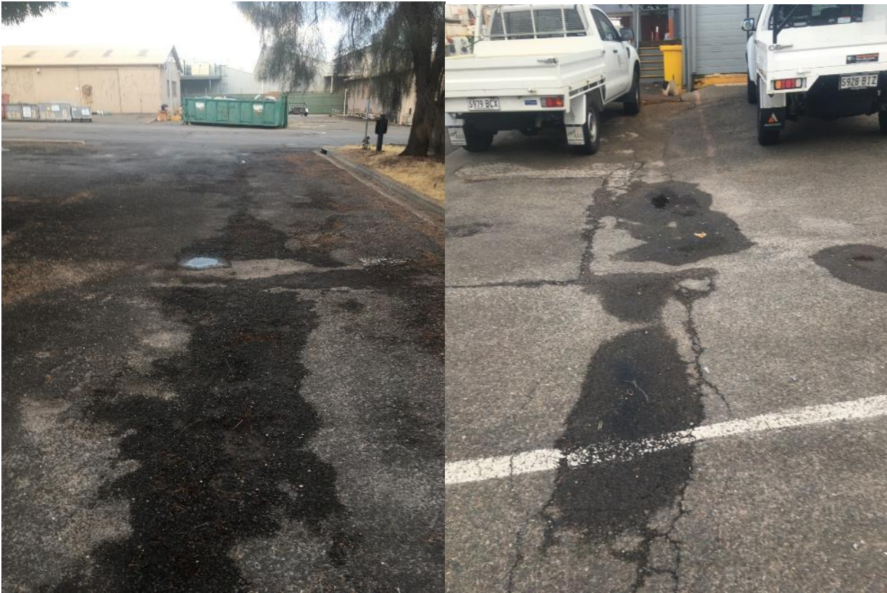
Figure 7 Example of full-thickness cracking, subsidence and potholing to main driveway and Car park area
