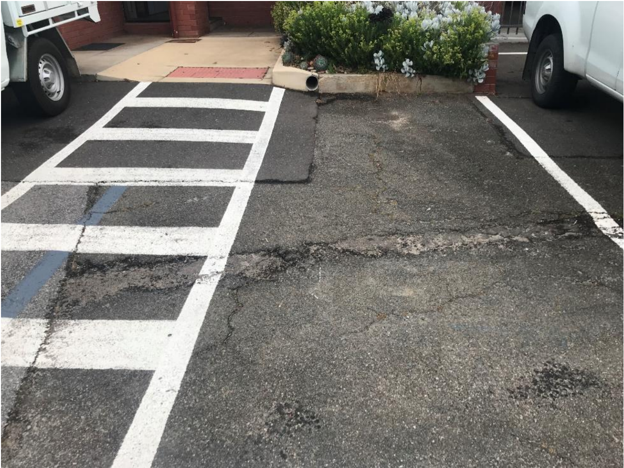
Figure 9 Example of cracking around pedestrian walkways
