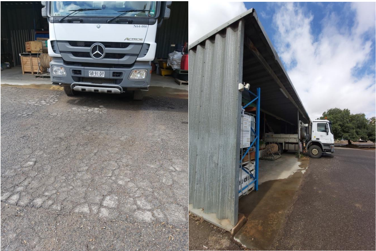
Figure 8 Broken and degraded pavements to the loading areas of the rear side of the truck store.
