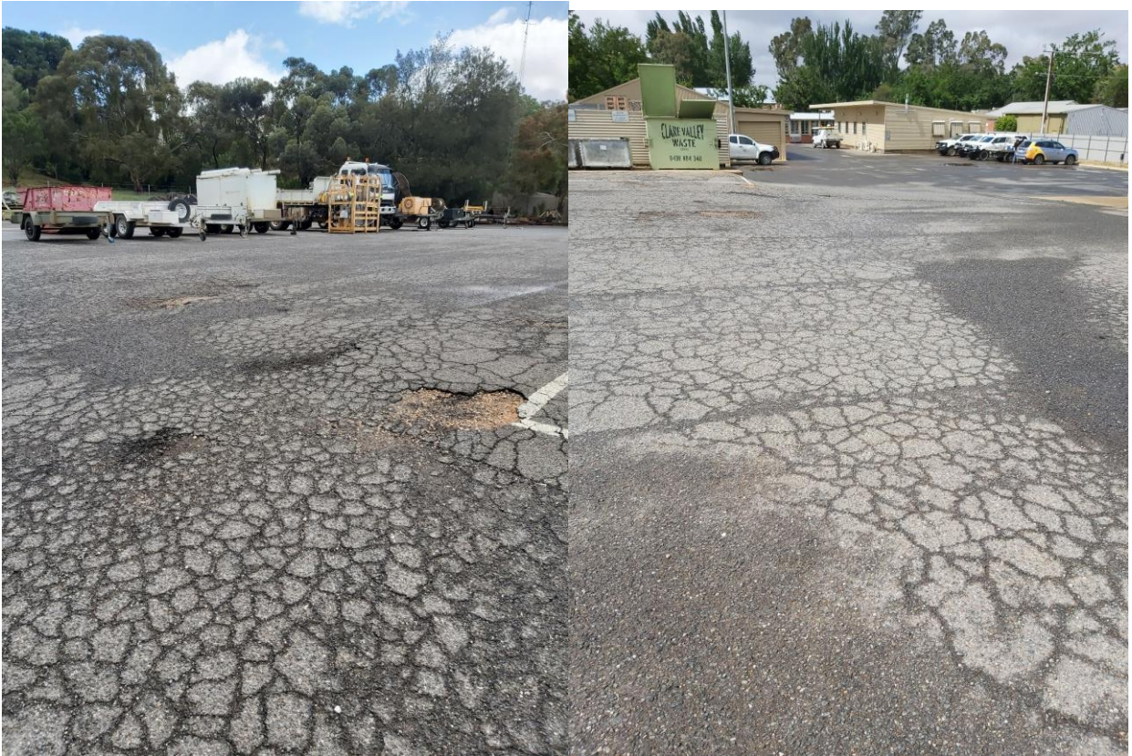
Figure 5 Examples of large areas of bitumen to the rear of the yard and heavy vehicle driveways in very poor condition with full-thickness cracking, potholing and subsidence.
