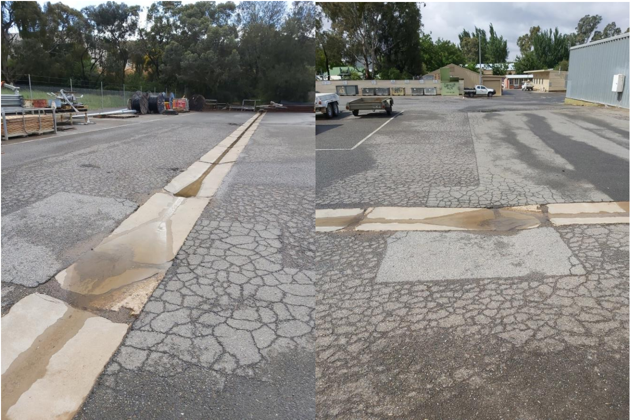
Figure 7 Examples of full-thickness cracking and breakdown of concrete drain and heavy vehicle driveway
