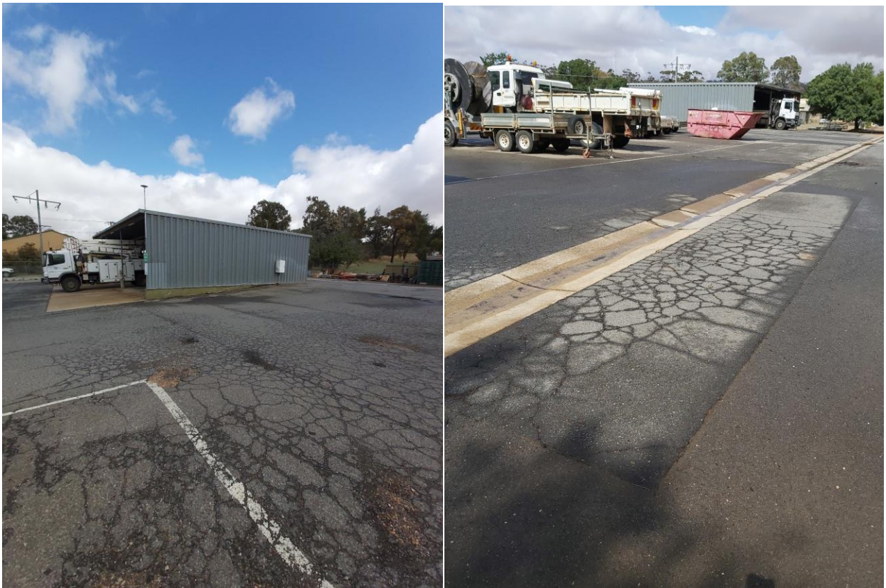
Figure 6 Examples of large areas of bitumen to the rear of the yard and heavy vehicle driveways in very poor condition.
