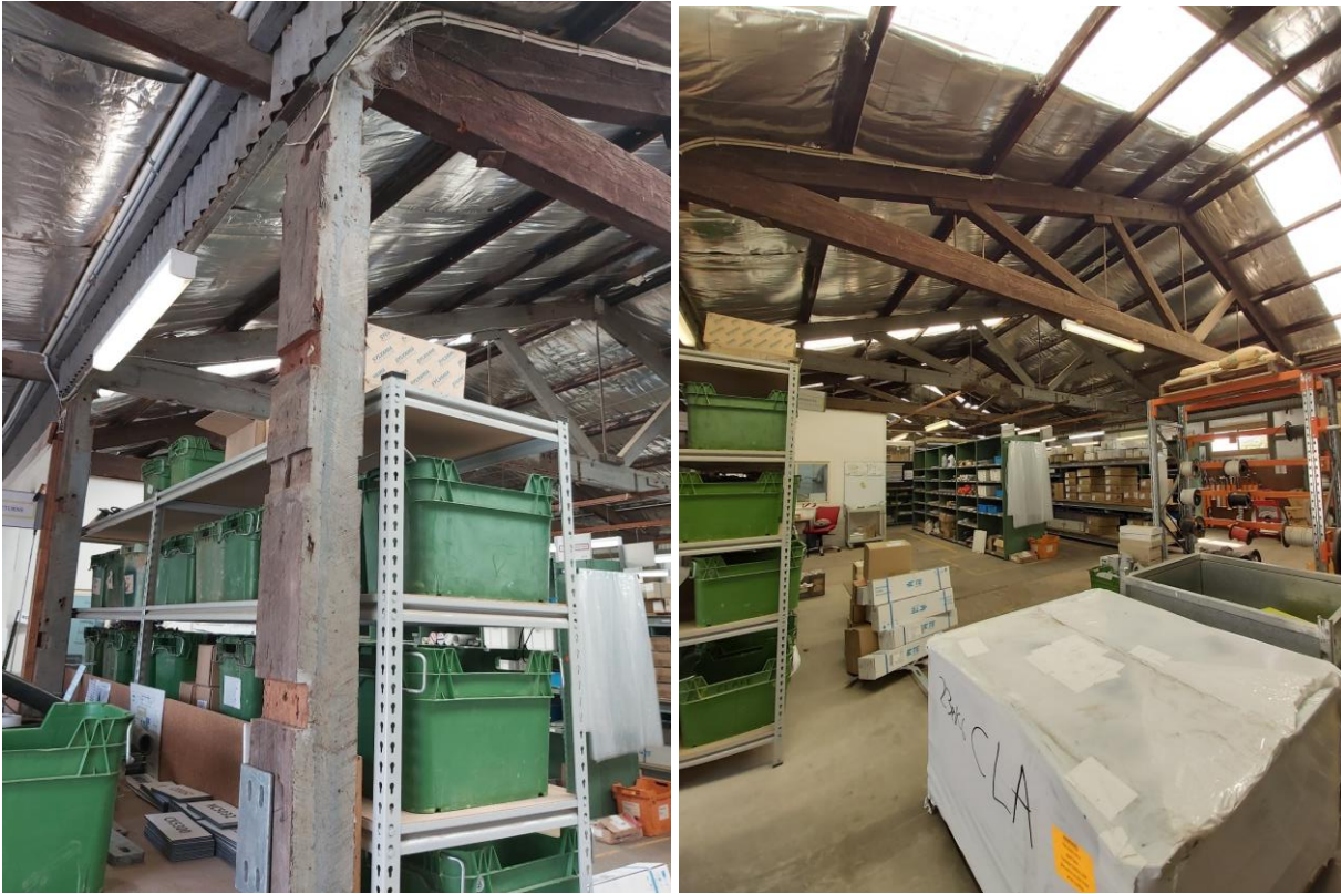
Figure 13 Inside the workshop building, showing the aged working arrangements including original Jarrah columns and trusses starting to show signs of cracking, height restrictions to operations and lack of effective insulation
