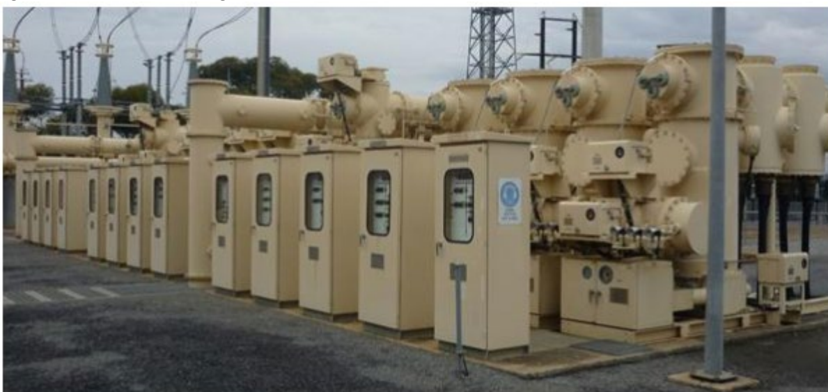
Figure 3: Present 66kV GIS configuration
