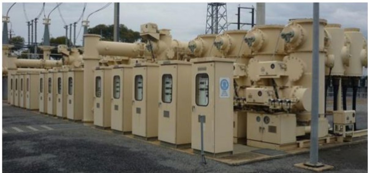
Figure 3: Present 66kV GIS configuration
