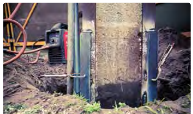
Image 20.2: Steel plating of a Stobie pole
