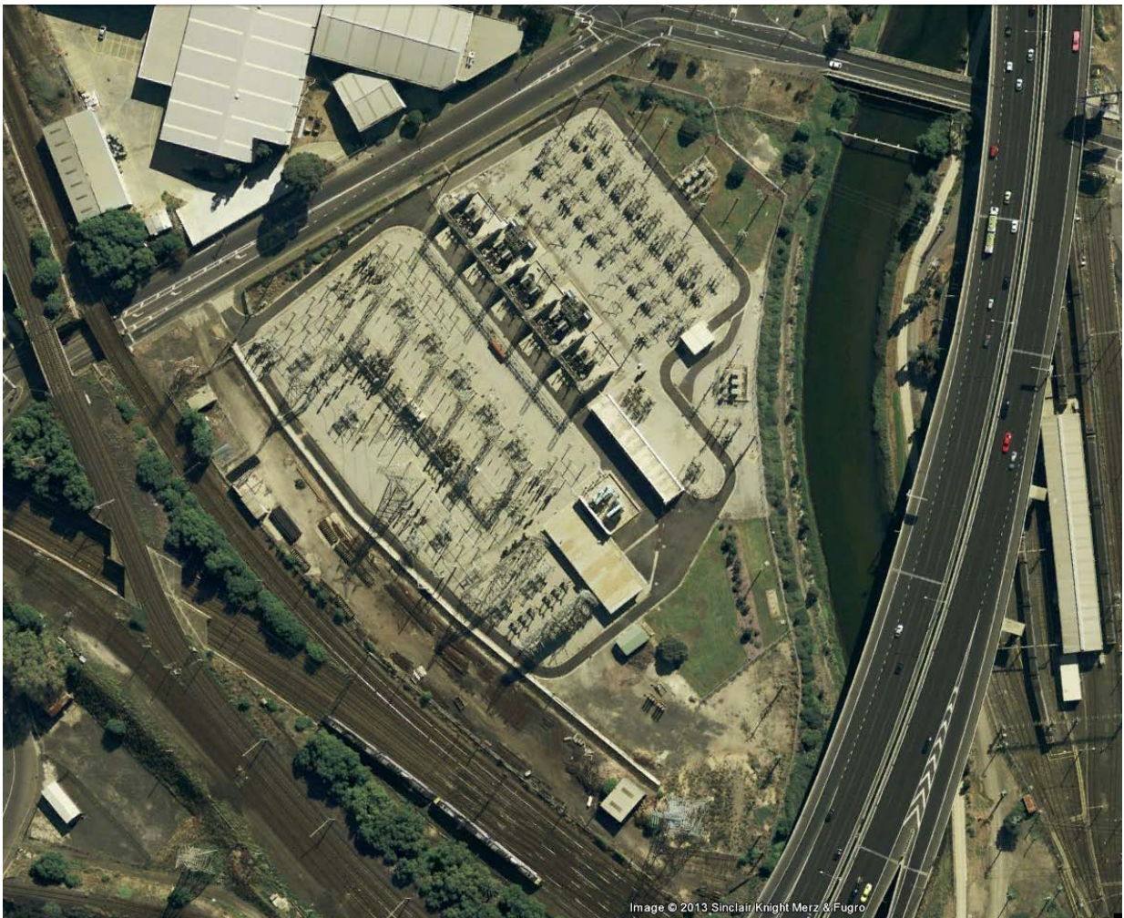
Figure 2: Aerial view of WMTS
