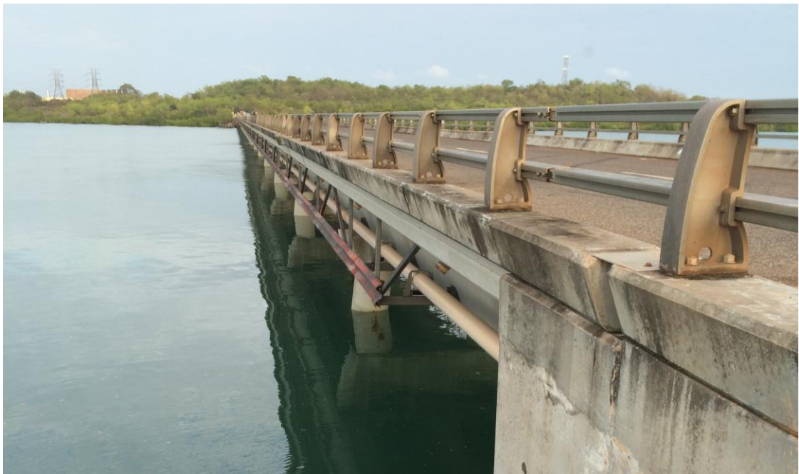
Figure 1: Channel Island Lateral - Channel Island Bridge Crossing (Note: Channel Island Power Station visible in left background)
