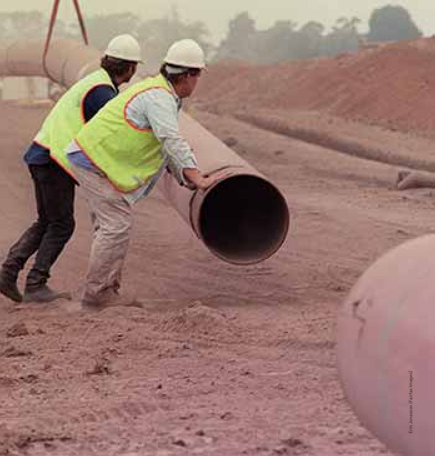
Laying of new gas pipeline
