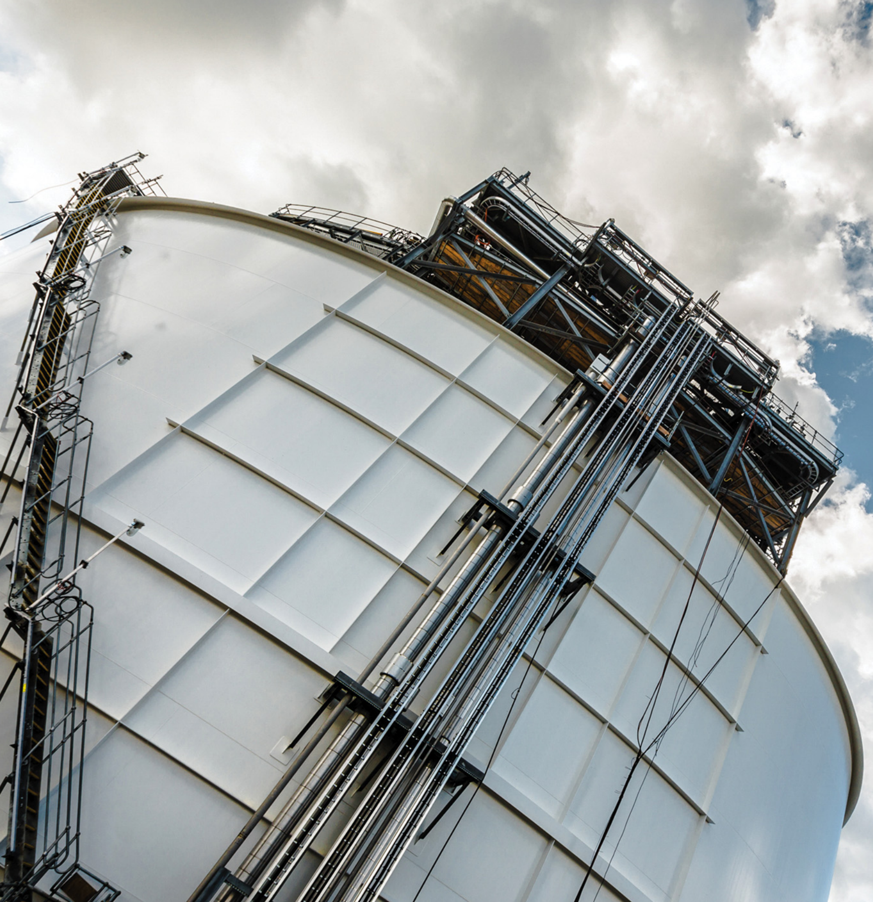
Newcastle LNG storage facility (image courtesy AGL Energy)
