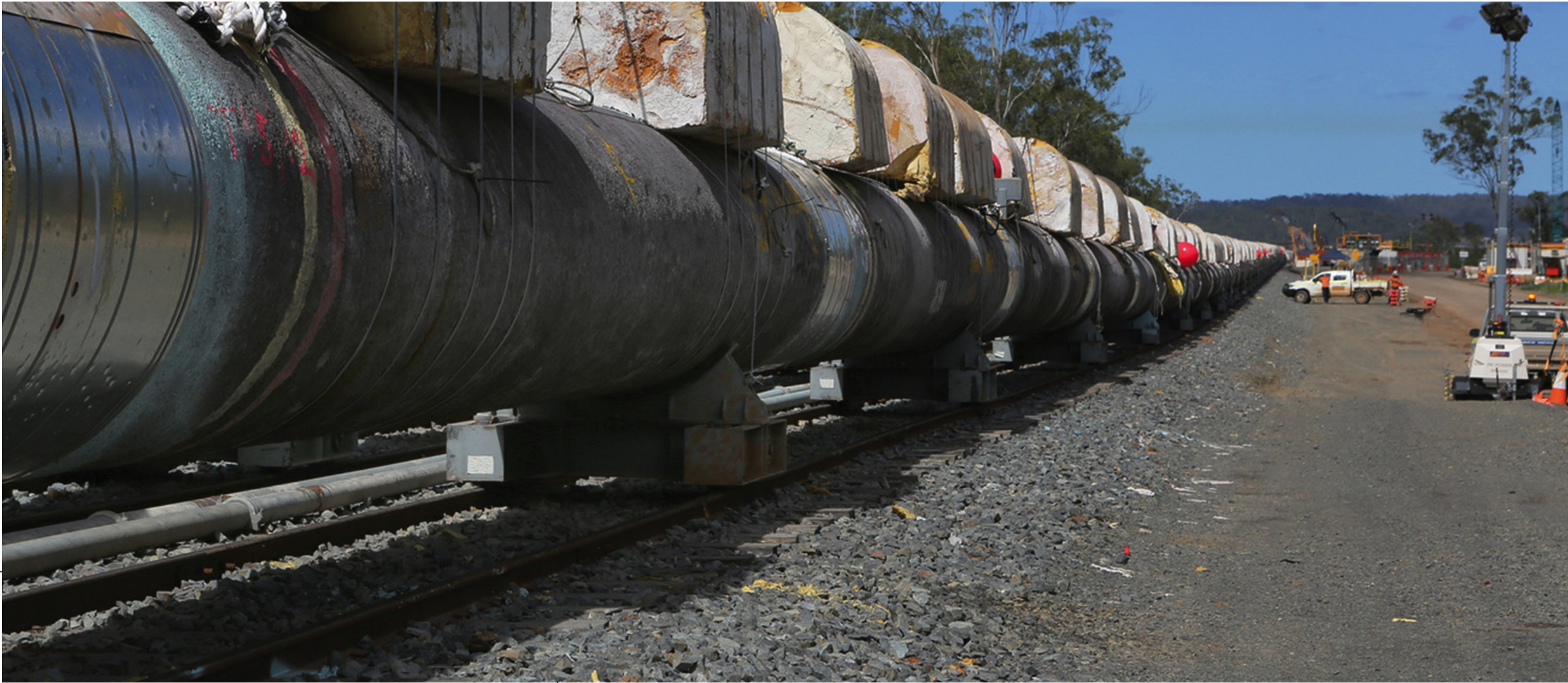
Construction of the Wallumbilla–Gladstone Pipeline (image courtesy of BG Group)
