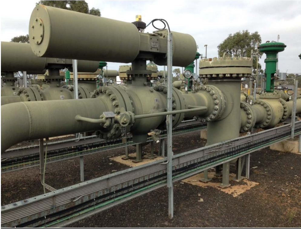
Regulator Run, Slam Shut Valve and filter
