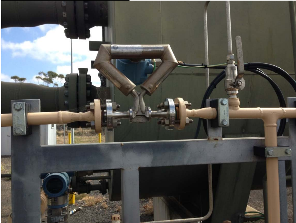
Heater Fuel Gas Flow Meter
