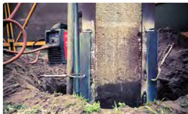
Image 20.2: Steel plating of a Stobie pole
