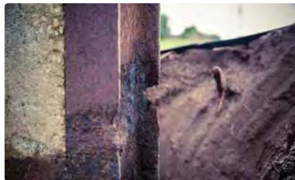
Image 20.2: Steel plating of a Stobie pole
