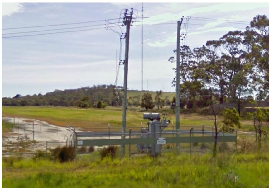
Figure 1: HV regulator installed adjacent to tidal flood plain
