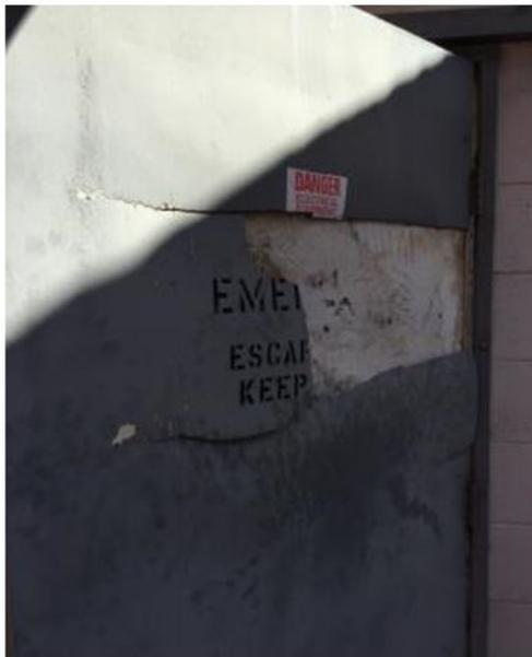
Figure 2 - Poor condition building type substation fire door
