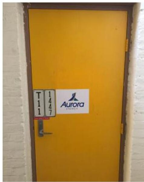
Figure 3 - New fire door which compliant with current building codes
