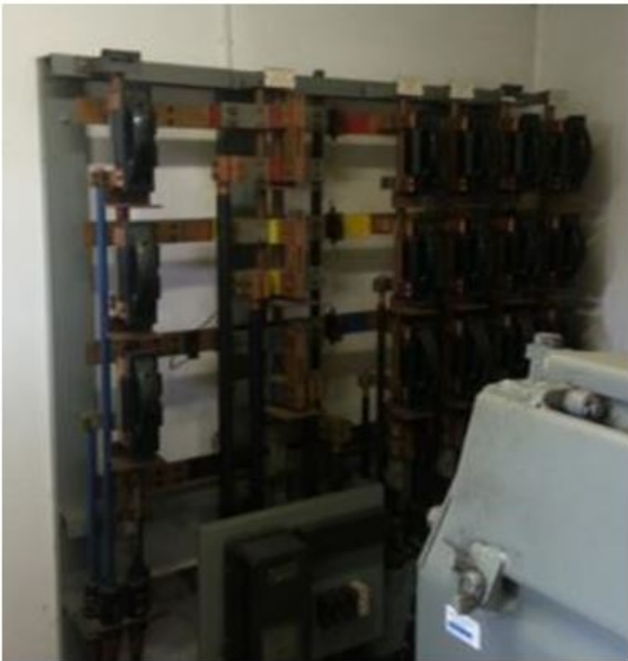
Figure 4 - Exposed live front board inside of a building type substation
