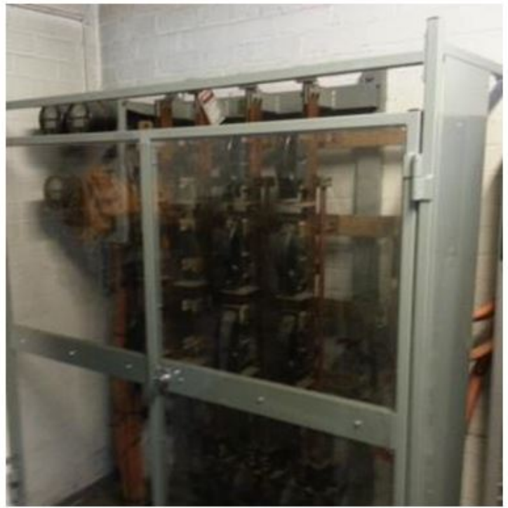
Figure 5 - Live front board covered up with Perspex enclosure
