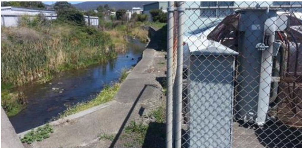
Figure 1 - Unbundled transformer next to waterway
