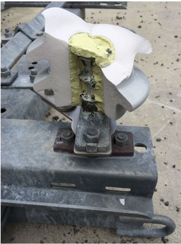
Figure 2: Porcelain insulator pin that has failed, as a result of steel corrosion.
