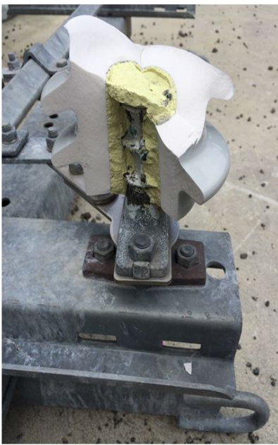
Figure 2 ABS porcelain insulator pin that has failed, as a result of steel corrosion.
