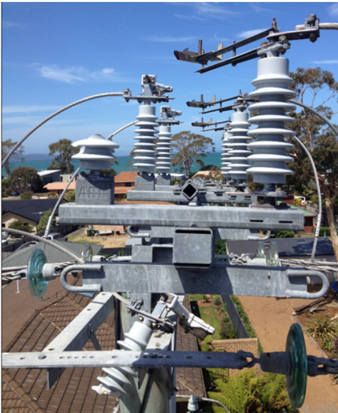
Figure 1: Damaged ABB air break switch.
