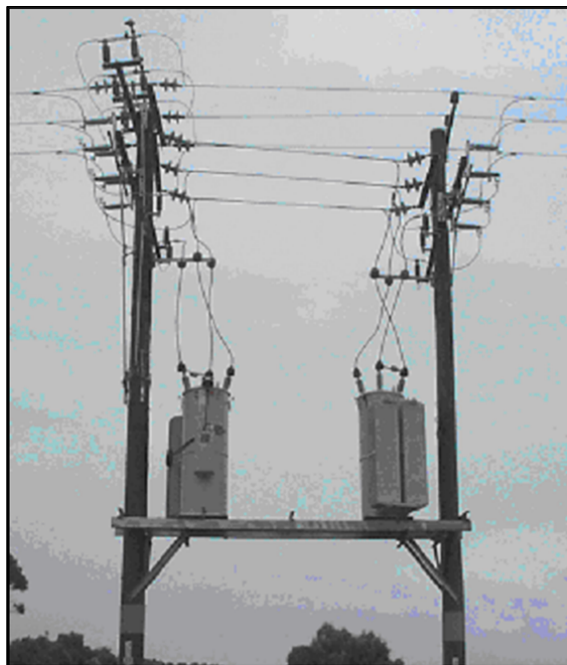
Figure 6: Typical three phase HV regulator site
