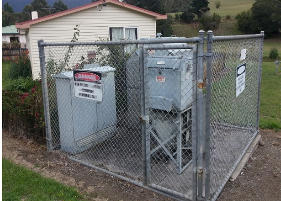
Figure 5 – Fence type substation (1967)
