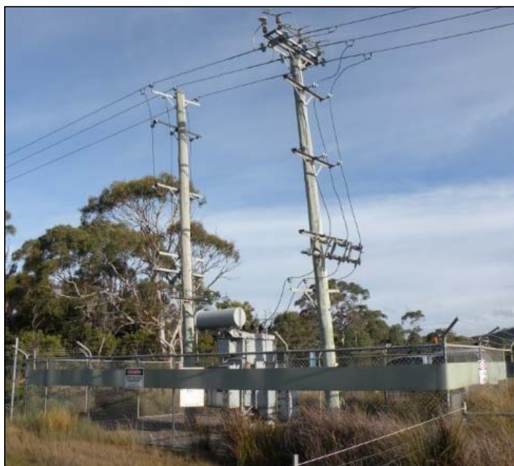
Figure 6: Typical three phase HV regulator site
