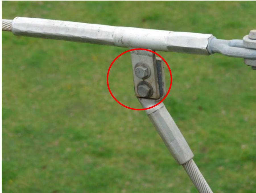
Figure 9: Dead end assembly with inadequate rating
