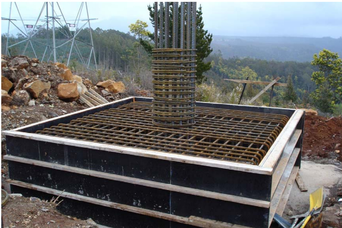
Figure 4 - Example of reinforcing steel in concrete foundation
