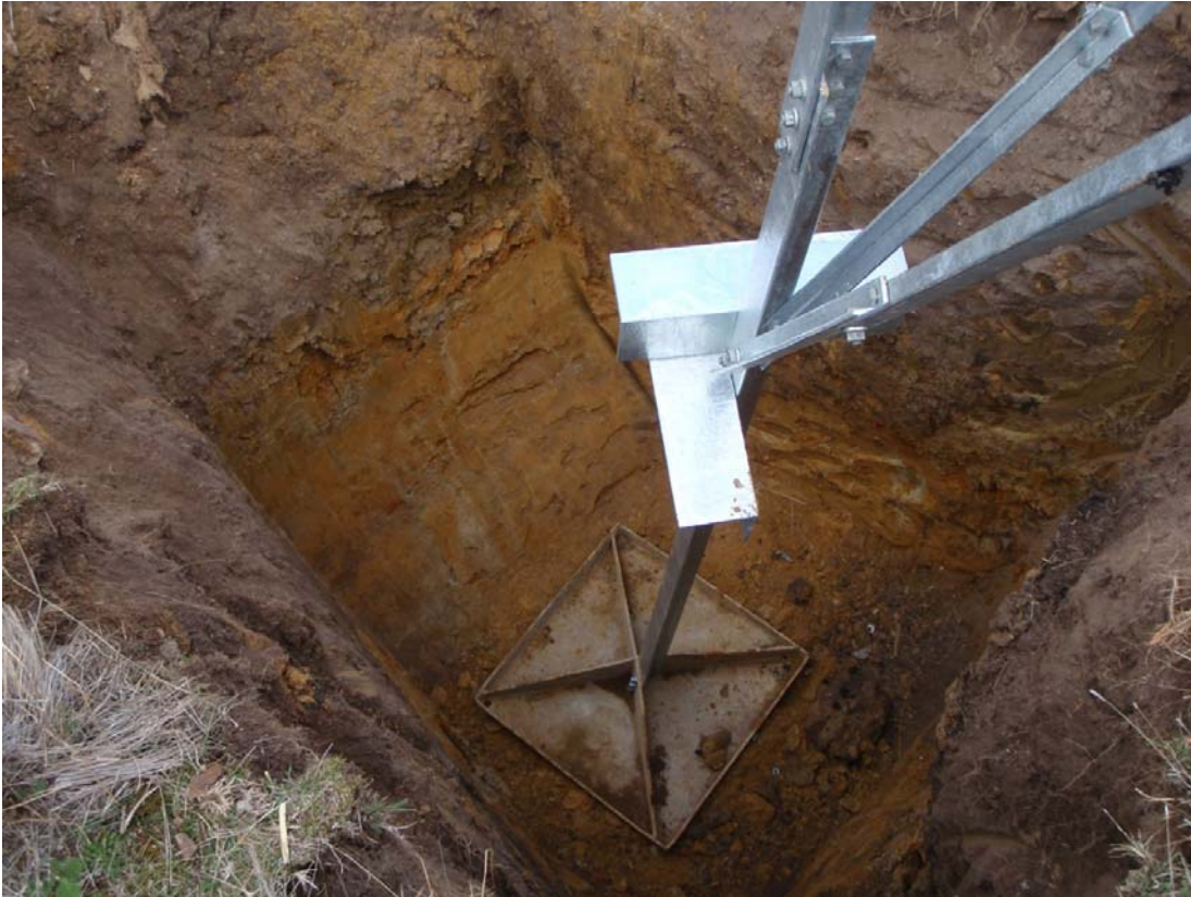
Figure 3 - Steel plate foundation example
