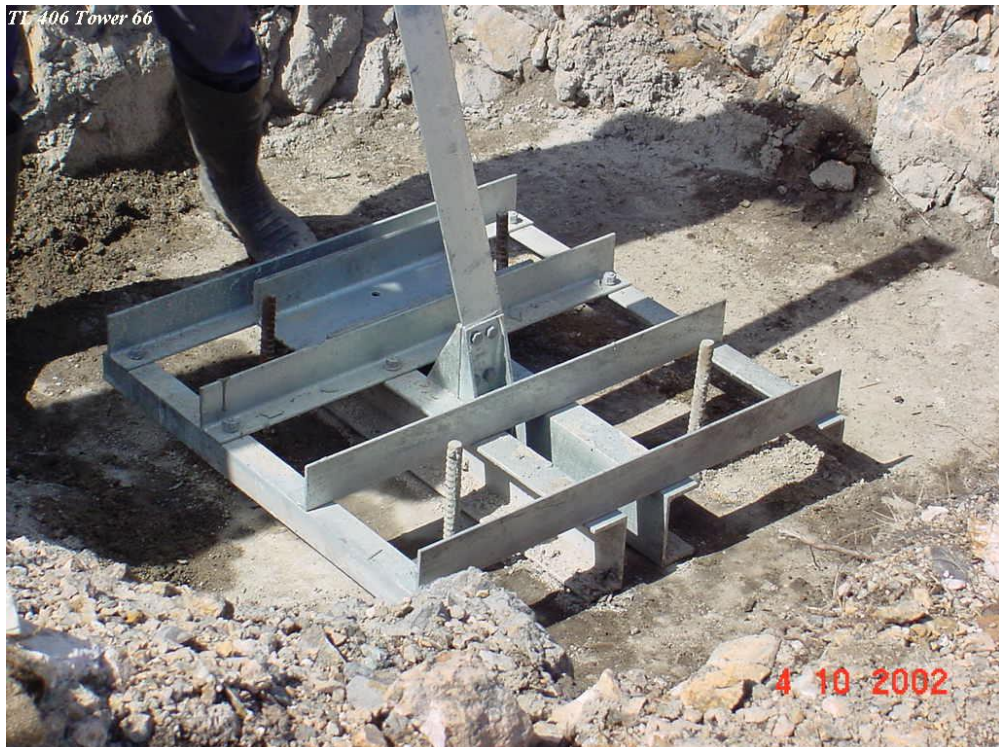
Figure 2 - Mini-grillage steel foundation example
