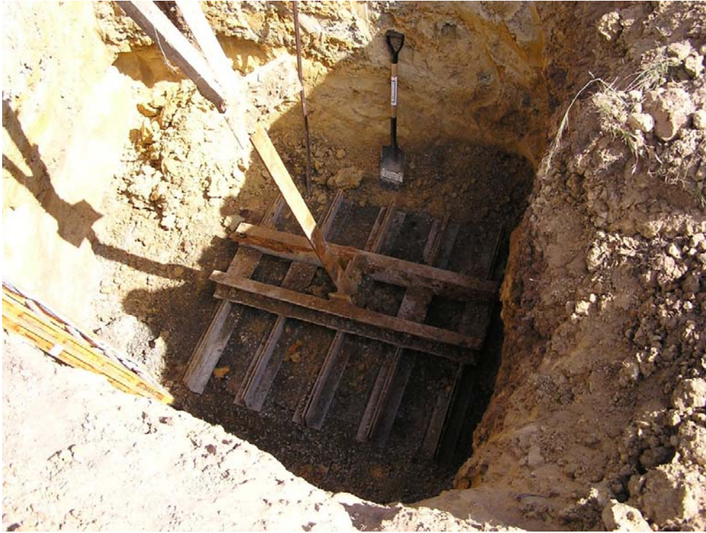
Figure 2 - Mini-grillage steel foundation example
