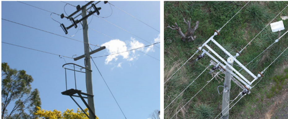
Figure 2: The same pole seen from the ground and from the air
