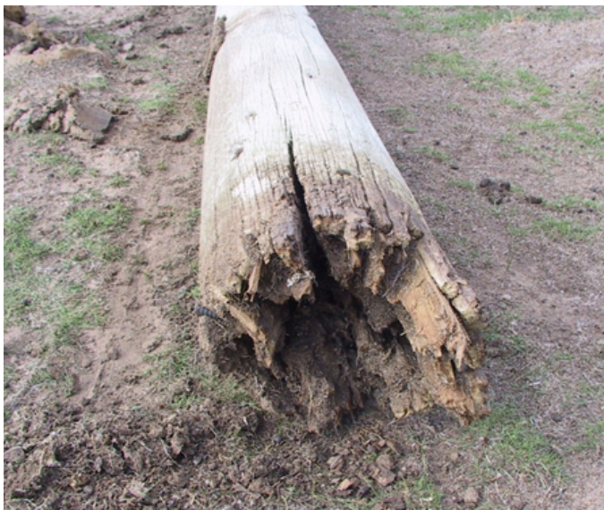
Figure 2: Wood pole that has failed in service
