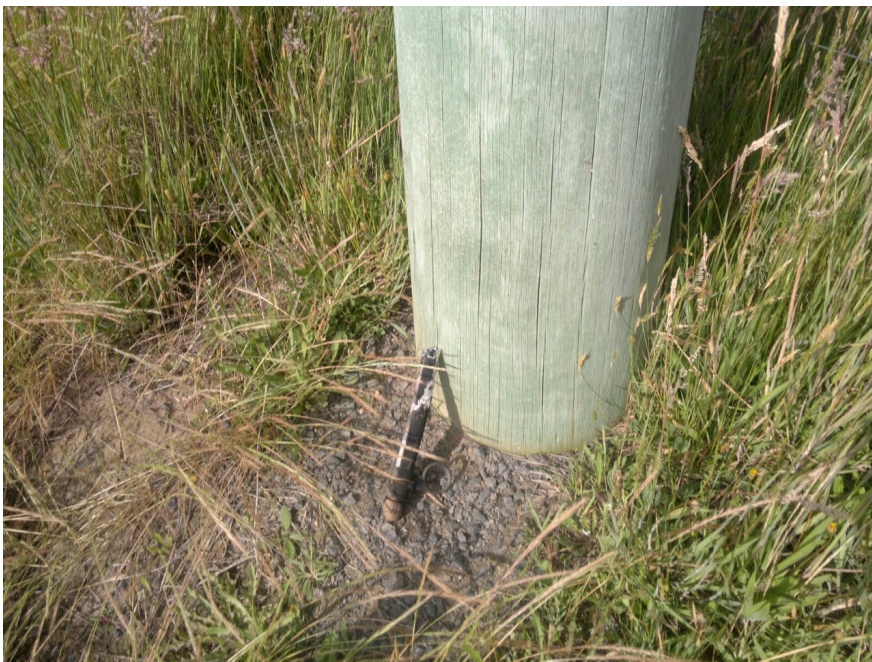
Failed EDO fuse tube
