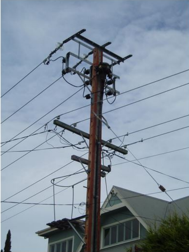
Figure 1 - High voltage cast iron cable termination
