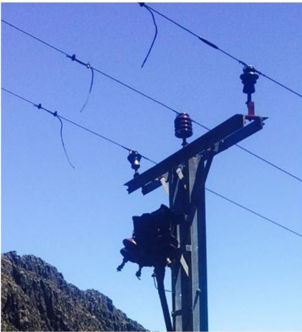
Figure 2 - HV pothead catastrophic failure
