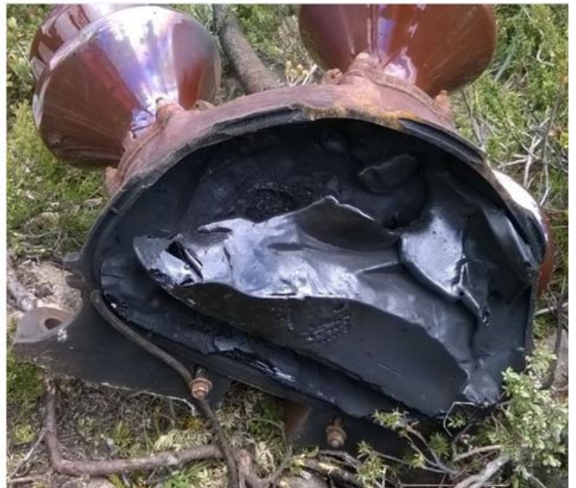
Figure 3 – High voltage cast iron cable termination failure.
