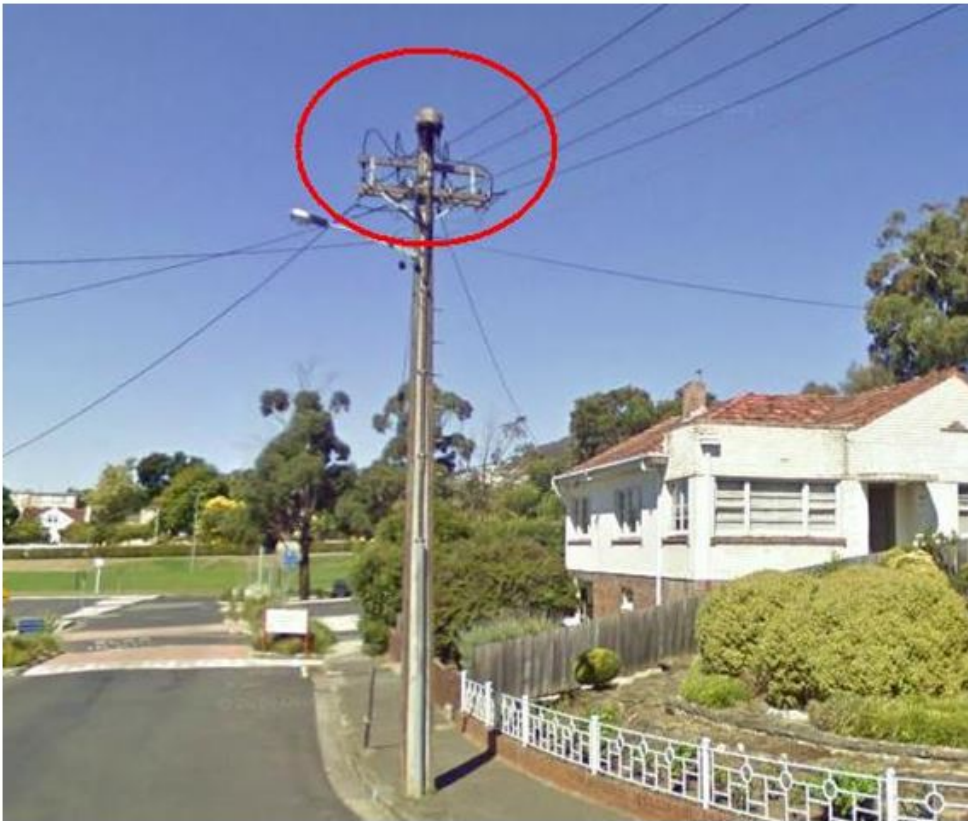
Figure 1: Low voltage cast iron cable termination
