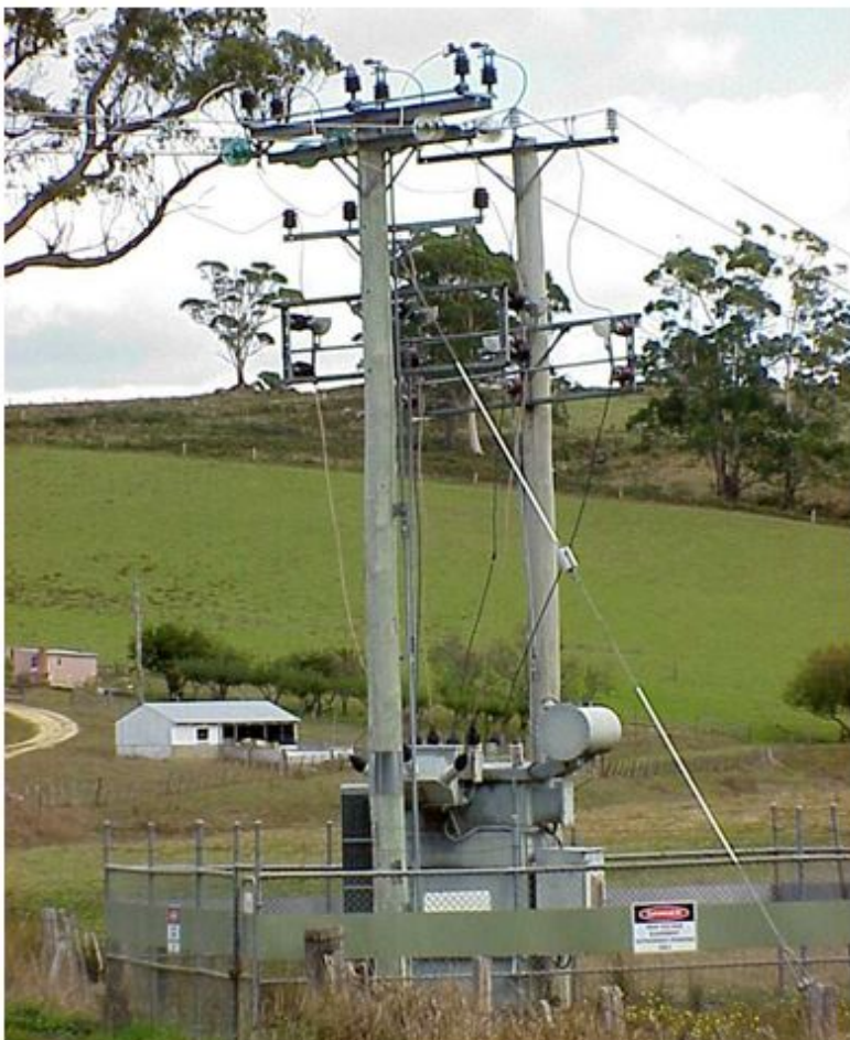
Figure 1 - Typical ground mounted regulator
